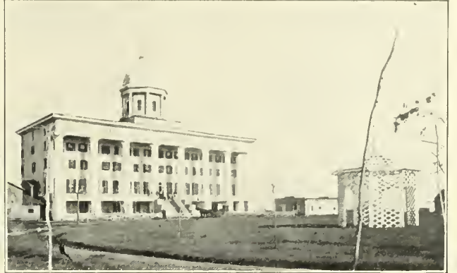
CHESAPEAKE HOSPITAL, HAMPTON, VIRGINIA
