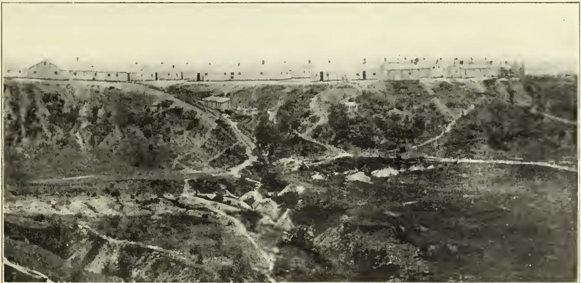
THE CHIMBORAZO HOSPITAL, RICHMOND, VIRGINIA
