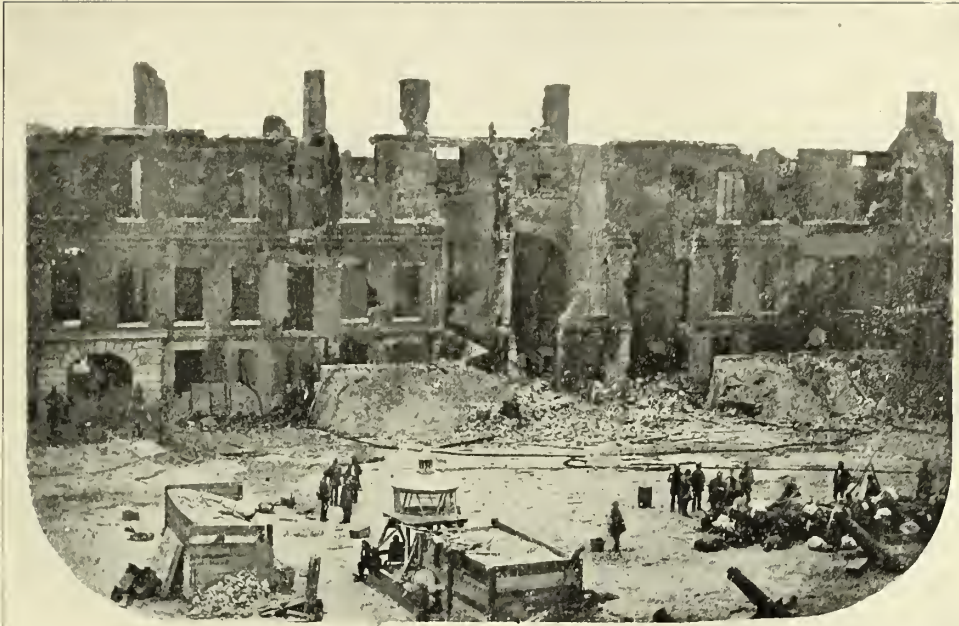
INTERIOR FACE OF GORGE.
