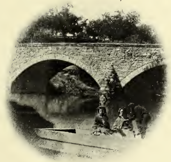
AT ANTIETAM BRIDGE
