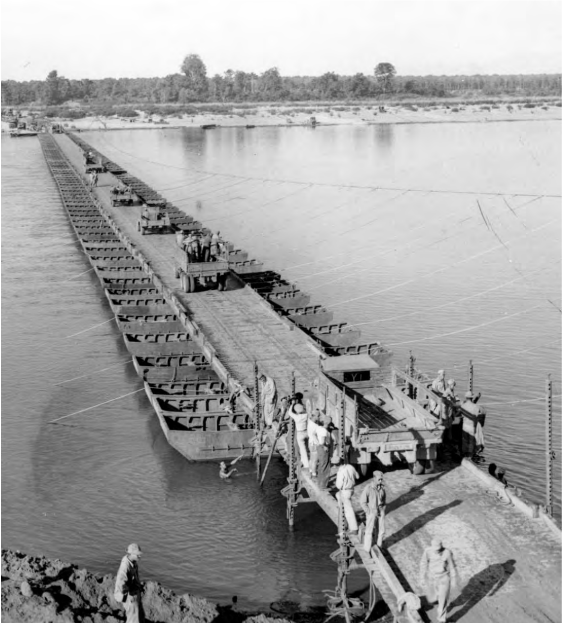
U.S. SERVICES OF SUPPLY TRUCK CONVOY starting across a temporary ponton bridge just after its completion in 1944. Built across the treacherous Irrawaddy River, this bridge was approximately 1,200 feet long and served as a link in the Ledo Road for the combat troops and supply vehicles. When the torrential rains ceased a permanent structure was built to handle the tremendous loads of the convoys going to China.
