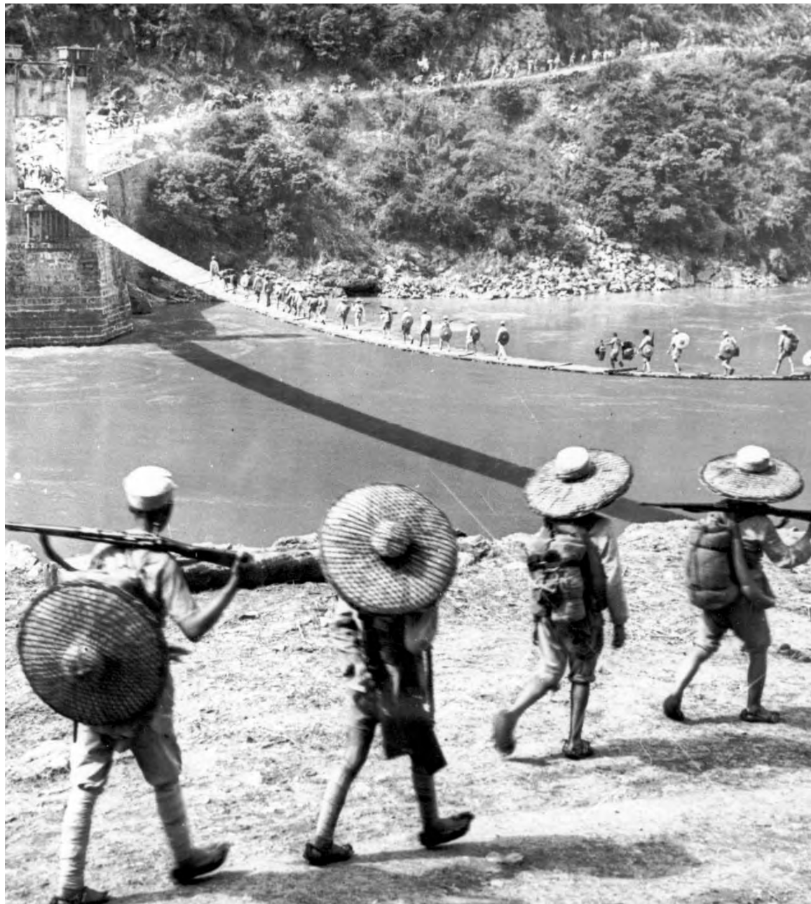
CROSSING THE SALWEEN RIVER, July 1944. The temporary suspension bridge was built to replace the permanent bridge here which was blown up in 1942 by the Chinese as a defense measure against the Japanese advance. While Allied forces advanced on Myitkyina, Chinese troops crossed the Salween River from the east. The two forces met at Teng-chung in September 1944, establishing the first thin hold in northern Burma.
