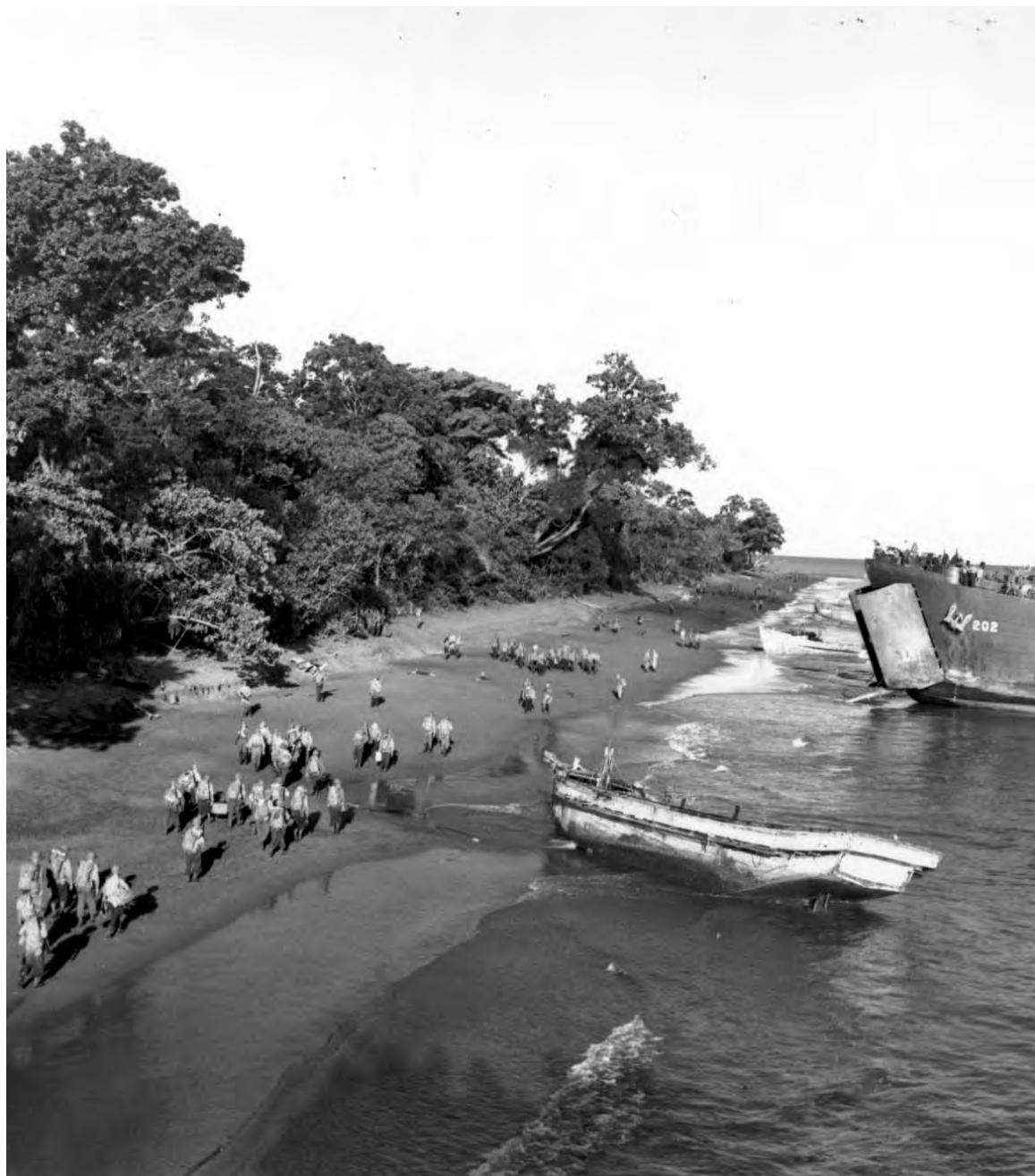
INFANTRYMEN MOVING ALONG THE BEACH at Cape Sansapor on 31 July; portion of LST in right background. The landings here were unopposed and the construction of new airfields began at once. By this move a large number of the enemy were bypassed and forced to begin an immediate withdrawal to the southwest coast.
