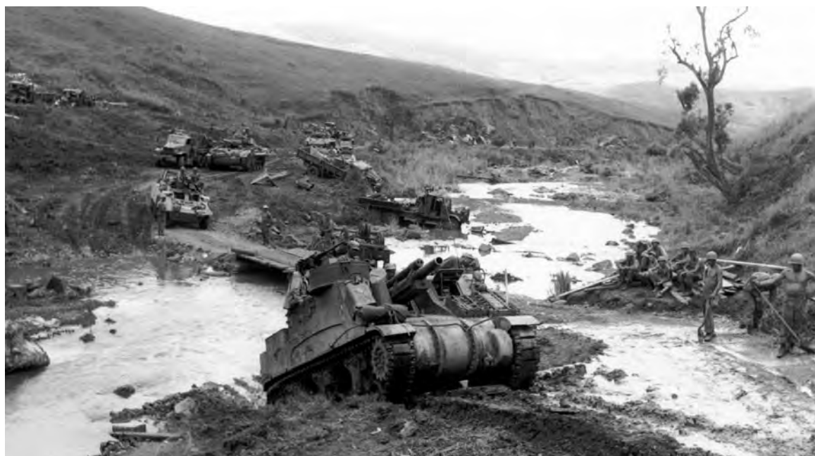
VEHICLES FORDING A RIVER in northern Luzon while engineer troops work on the road; in foreground is a 105-mm. howitzer motor carriage M7. Note destroyed enemy vehicles along road and in stream (top). A bulldozer and a medium tank help another medium tank which has struck a road mine (bottom).
