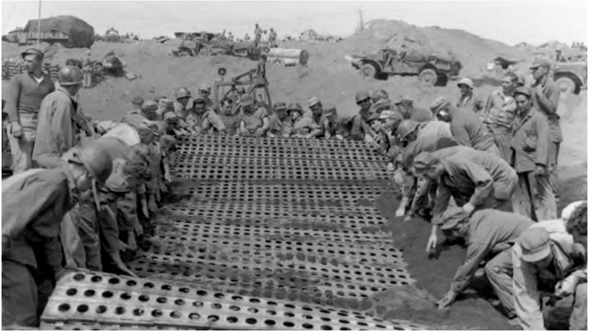
STEEL MATTING BEING LAID on the beach at Iwo Jima to facilitate the unloading of heavy equipment over the sand. Both on the beaches and inland the loose volcanic soil made the movement of vehicles extremely difficult. Trucks bogged down and supplies soon piled high on the beach.
