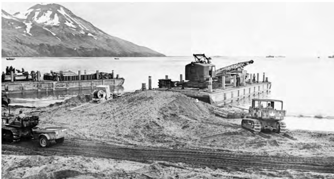
HEAVY BARGE, loaded with a crane and other heavy machinery, in the Massacre Bay area on 31 May 1943, having been towed to shore by tugs. In order to get the crane off, it was necessary to make a sand ramp leading from the shore to the deck of the barge. Tractor at right is a 7-ton, high-speed tractor M2 (top). An oil and gas dump; at the left can be seen a motor pool (bottom). The battle for Attu ended on 30 May but mopping-up operations continued for several days.
