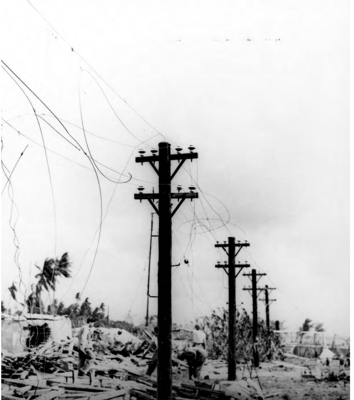
WRECKAGE OF A JAPANESE POWER INSTALLATION found on one of the islands in the Kwajalein Atoll on 31 January 1944. As a result of the air, naval, and artillery bombardment, the islands were greatly damaged. With exception of rubble left by concrete structures, there were no buildings standing; all those which had been made of any material other than concrete were completely demolished.
