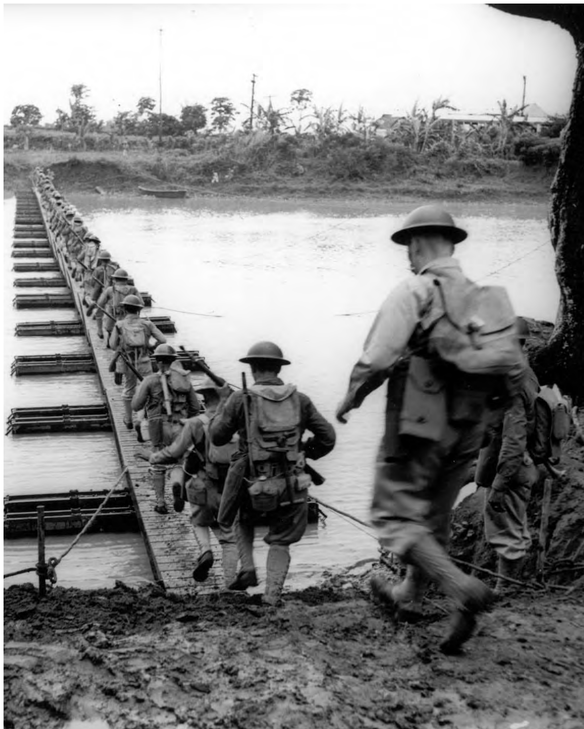
TROOPS CROSSING the newly constructed ponton bridge.
