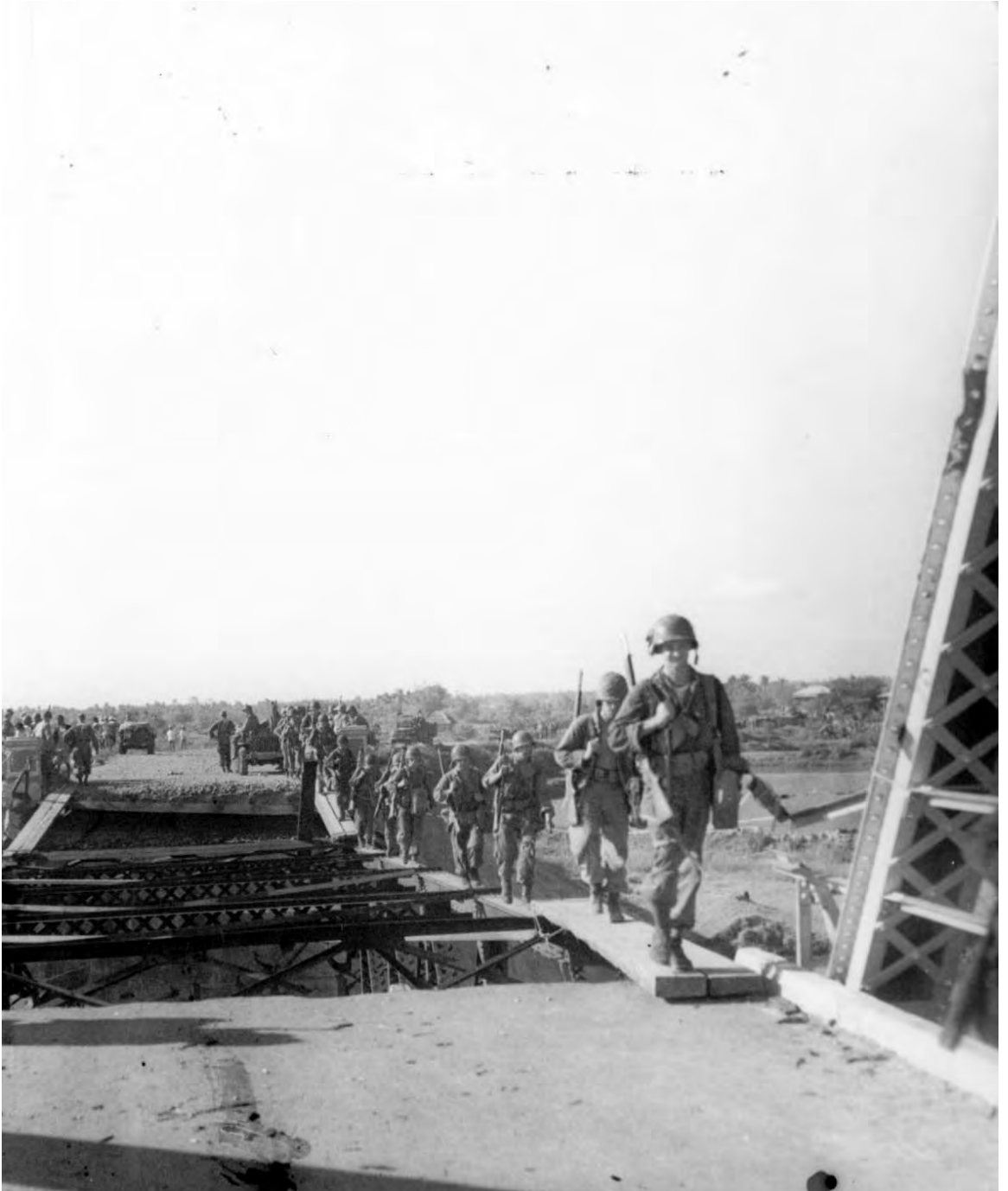
U.S. INFANTRYMEN CROSSING A DAMAGED BRIDGE as they advance inland from the beach. The advancing U.S. troops found the bridges destroyed. Some had been destroyed in 1942 during the Japanese conquest of the Philippines.
