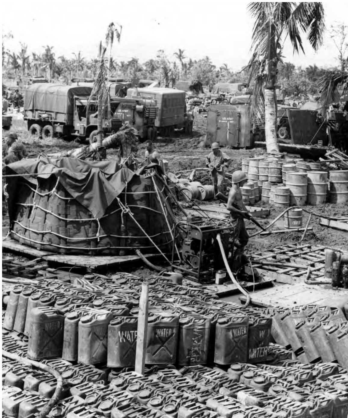
WATER SUPPLY POINT set up near a beach on Leyte, 21 October; note the collapsible water tank. By the end of the 21st, Tacloban, San Jose, Dulag, and two airfields were captured. Heavy fighting continued at Palo.
