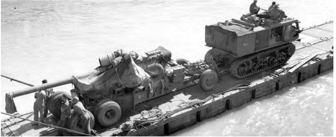
TRACTOR TOWING A 155-MM. GUN OVER A PONTON CAUSEWAY reaching from an LST to shore on Saipan. The tractor is a high-speed 18-ton M4 model; the 155-mm. gun M1A1 is mounted on an M1 carriage (top). A landing vehicle, tracked, provides a shady spot for a game of cards during a lull in the fighting; this armored amphibian LVT (A) (4) was the same as the LVT (A) (1) except for an M8 75-mm. howitzer turret which replaced the 37-mm. gun (bottom). On Saipan tanks and heavy artillery added the weight of their guns to renewed naval gunfire and aerial bombardment after the Battle of the Philippine Sea.
