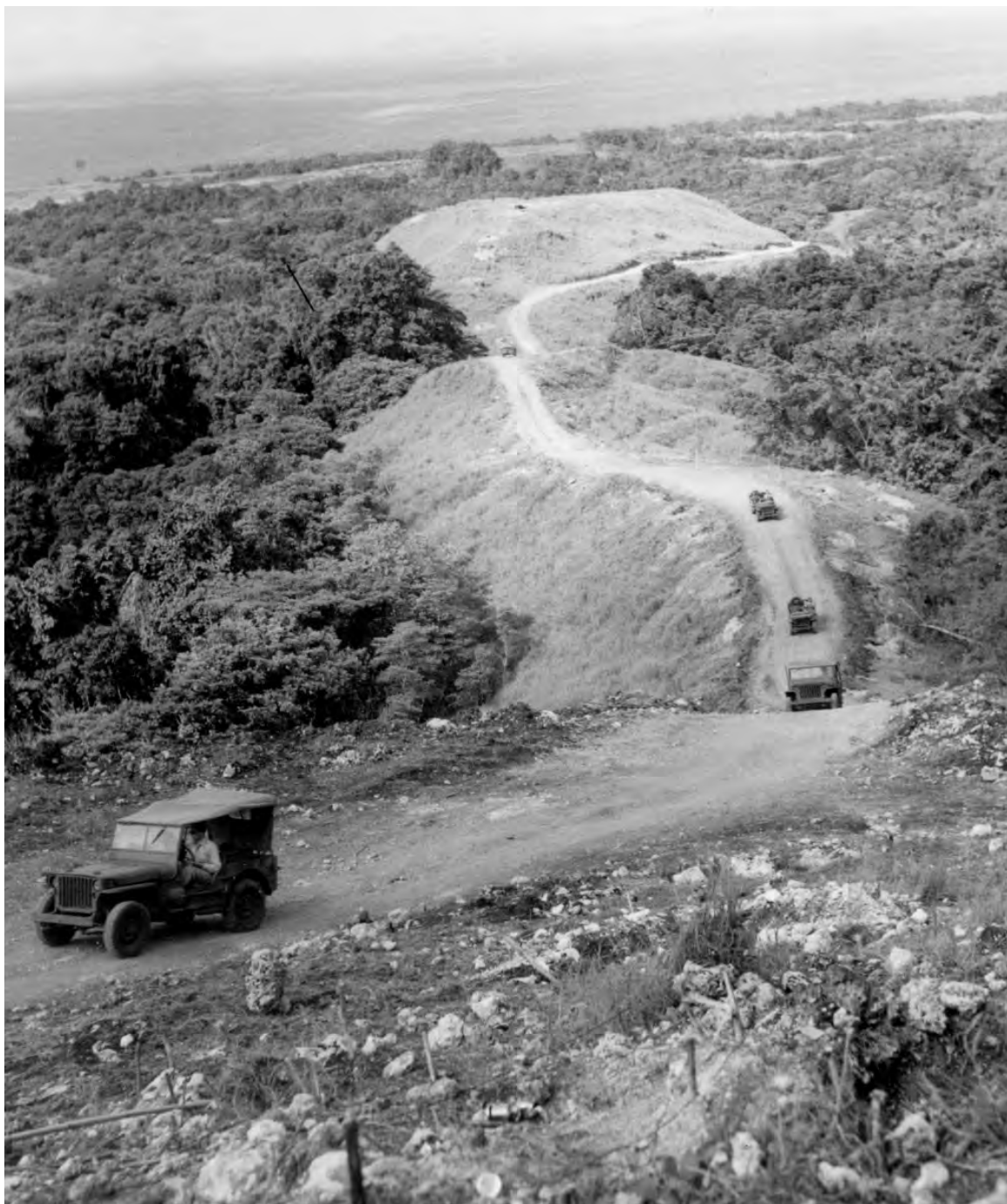
JEEPS ON NARROW TRAIL. This trail, having many grades approaching 40 degrees, was slick and dangerous after heavy rains and was of little use for heavier vehicles.
