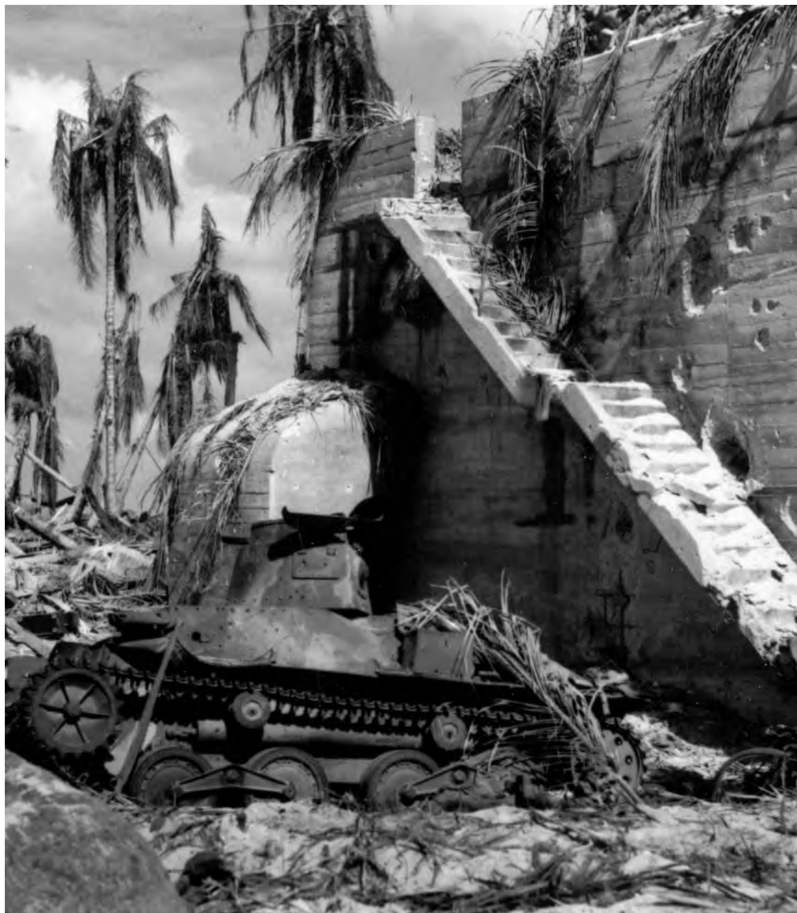
CAPTURED JAPANESE COMMAND POST with enemy tank in foreground. Shells and bombs had little effect on this reinforced concrete structure. Most of the command posts, ammunition dumps, and communications centers found here were made of reinforced concrete and were virtually bombproof. Powerful hand-to-hand infantry assault tactics were necessary to dislodge the enemy.
