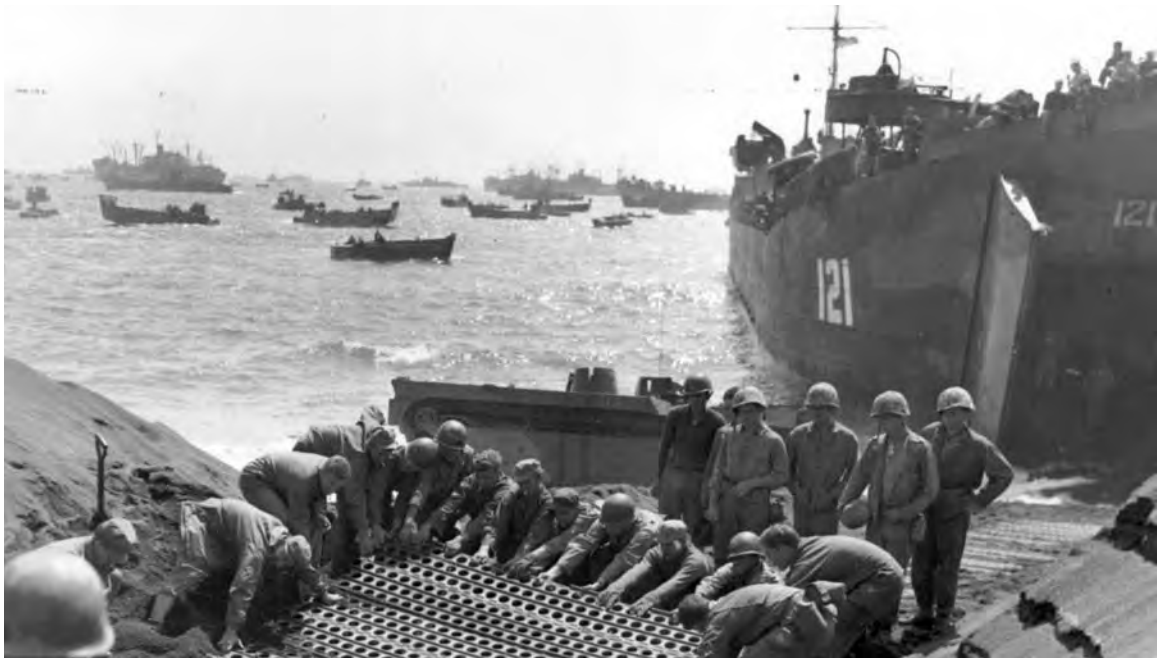
STEEL MATTING BEING LAID on the beach at Iwo Jima to facilitate the unloading of heavy equipment over the sand. Both on the beaches and inland the loose volcanic soil made the movement of vehicles extremely difficult. Trucks bogged down and supplies soon piled high on the beach.
