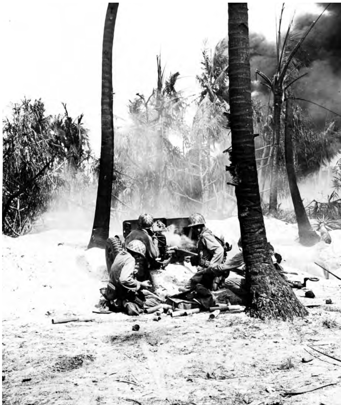
FIRING A 37-MM. ANTITANK GUN M3A1 at an enemy pillbox, 31 January. The operations on Roi, Namur, and Kwajalein consisted mostly of ferreting the enemy from his concrete pillboxes.
