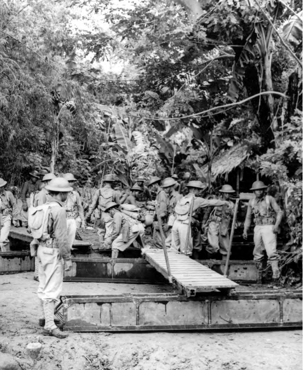
ENGINEER TROOPS stand ready to place sections of a ponton bridge in position during a river-crossing maneuver in the Philippines, 1941.
