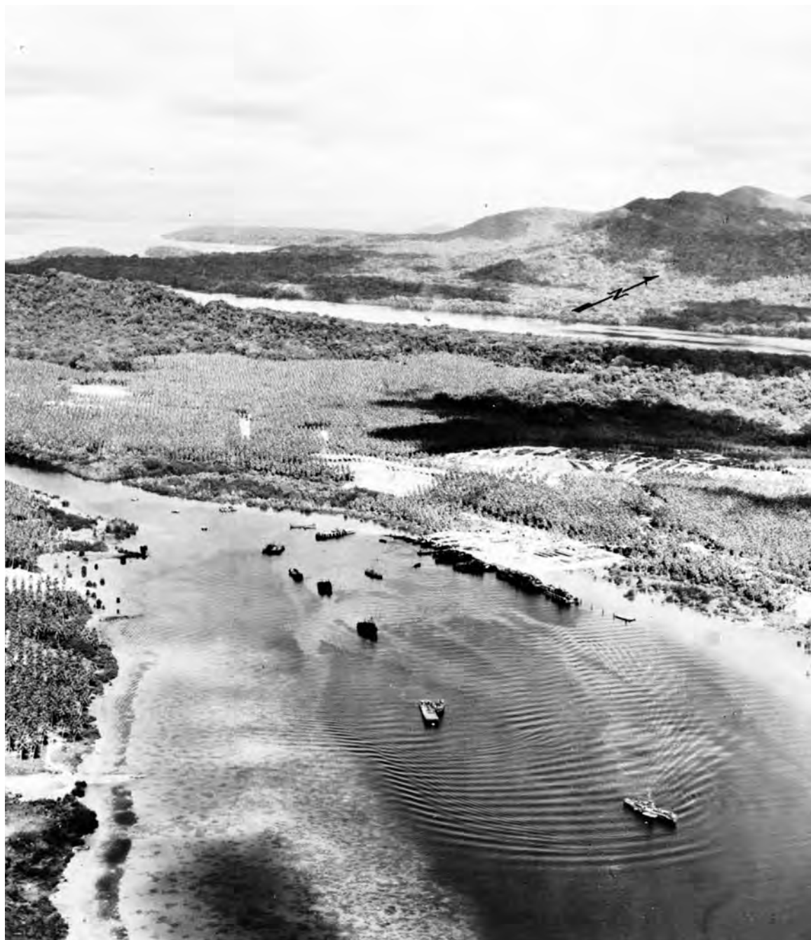
RENARD SOUND, separating the two airfields on Banika. Construction of roads, airfields, and boat bases began in February and by 15 April the first of the two airfields was ready for operation. The torpedo boat base at Lingatu (Wernham) Cove went into operation on 25 February.
