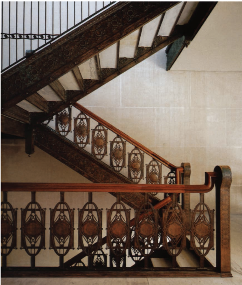
5. Louis H. Sullivan (1856–1924). One of two pairs of staircases for the Chicago Stock Exchange Building, 1893. Cast iron with electroplated copper finish. Sullivan was uniquely skilled at integrating utilitarian construction and elegant ornament. Purchase, Mr. and Mrs. James Biddle Gift and Emily Crane Chadbourne Bequest, 1972 (1972.50.1–4)
