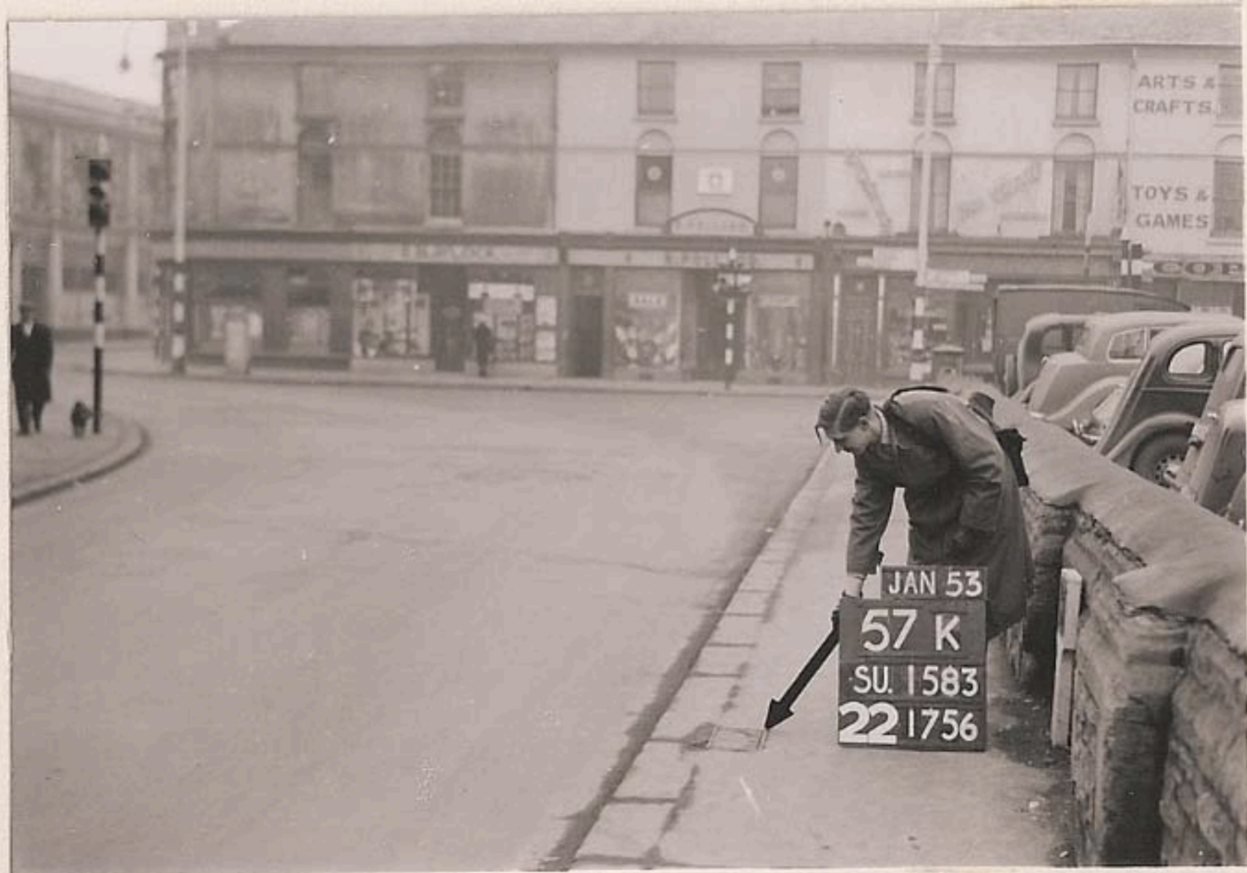
RP. 57K. SW. corner of hydrant cover, Victoria Road
