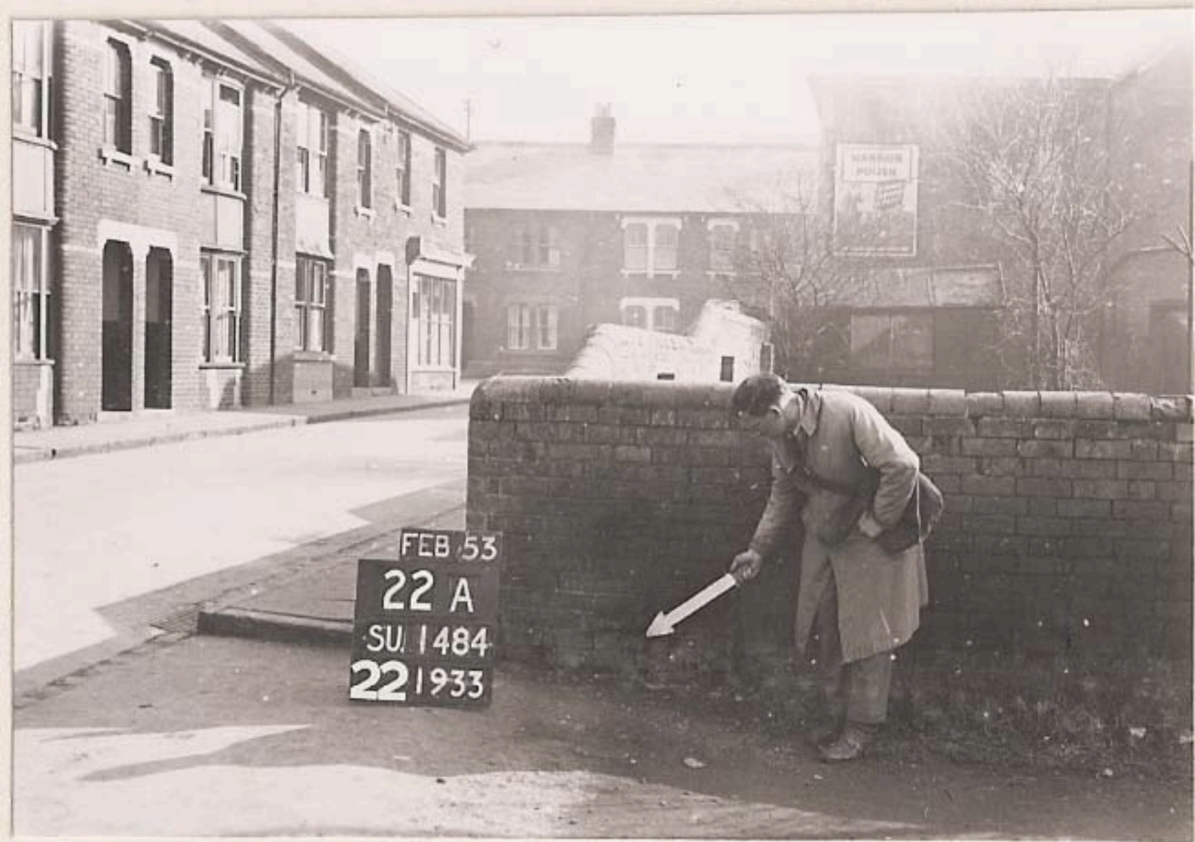
RP. 22A. Pipe Nail in wall at rear of No. 108 Albion Street.
