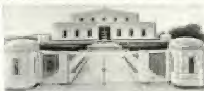
Builders of the U.S. Gold Storage Vault Doors at Fort Knox, Ky.
