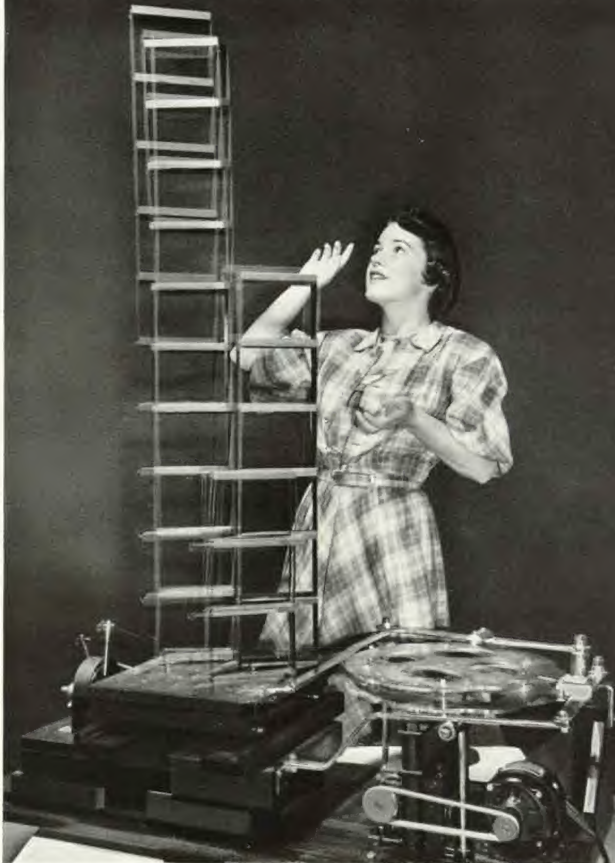
A Make-believe Quake Rocks Building Models, Showing What Happens in a Real Temblor Multiple images caught by the camera reveal how miniature skyscrapers whip back and forth on the shaking table in a demonstration at California Institute of Technology. Such tests help design safer structures.
