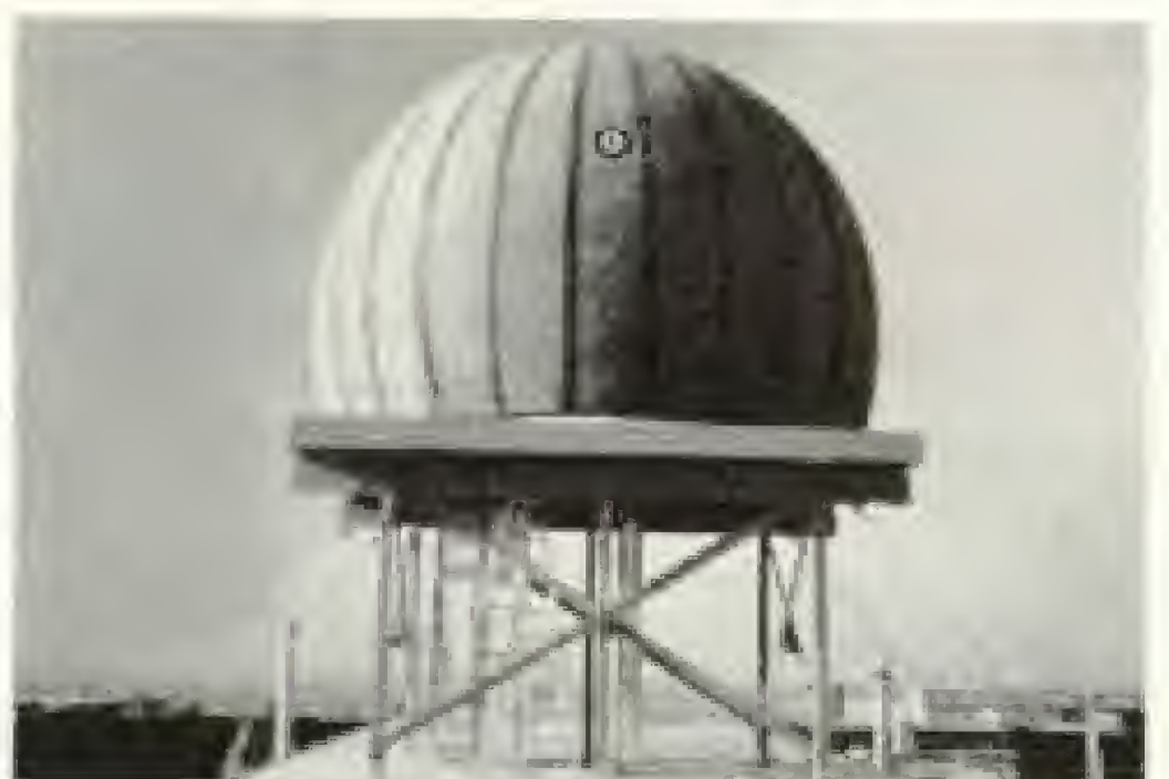
RUBBER IGLOO FOR RADAR. Strange domes like this protect radar antennas from Arctic storms.
