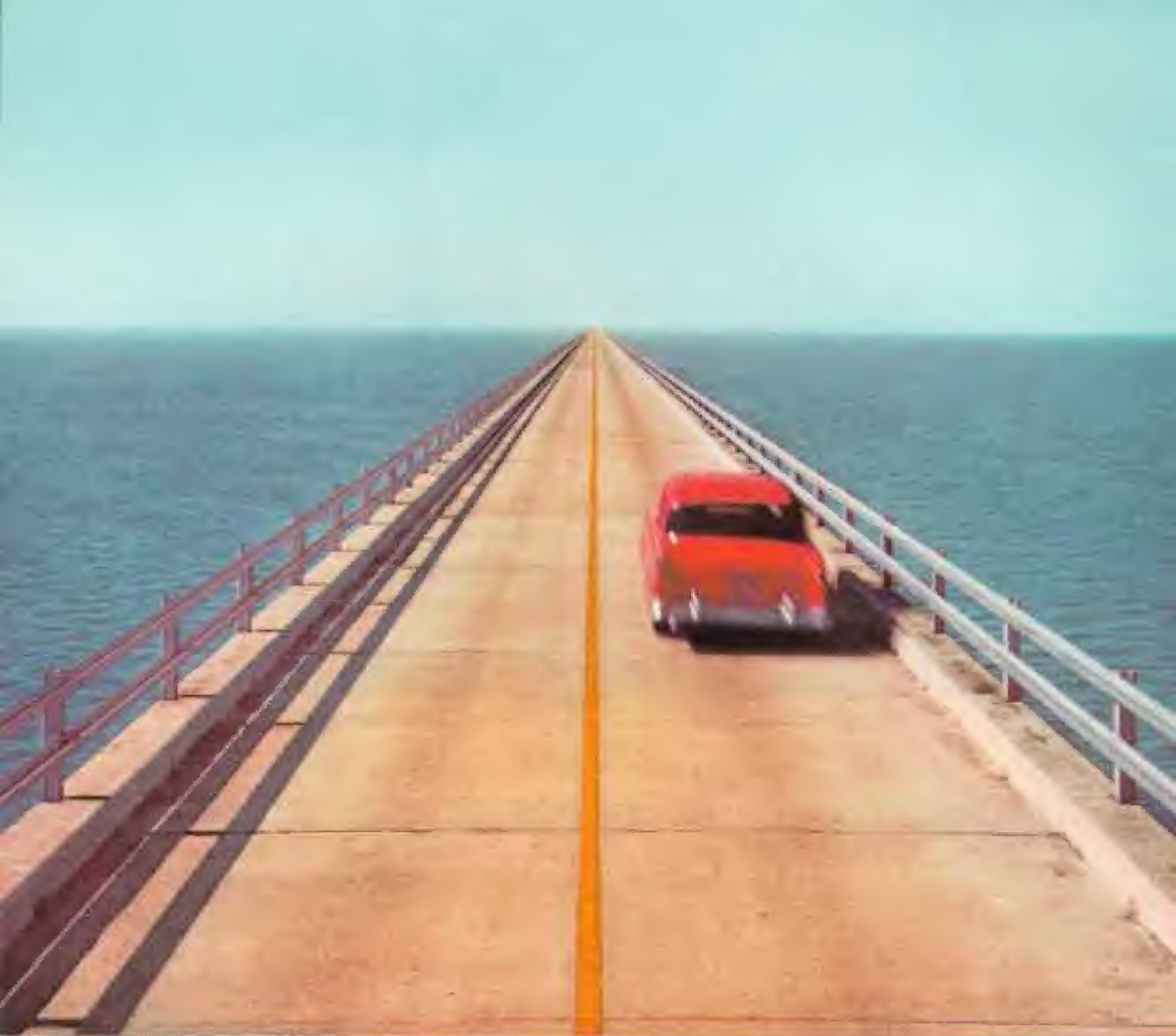
Seven-Mile Bridge on Florida's Key West County—one of America's longest open-water bridge crossings.
