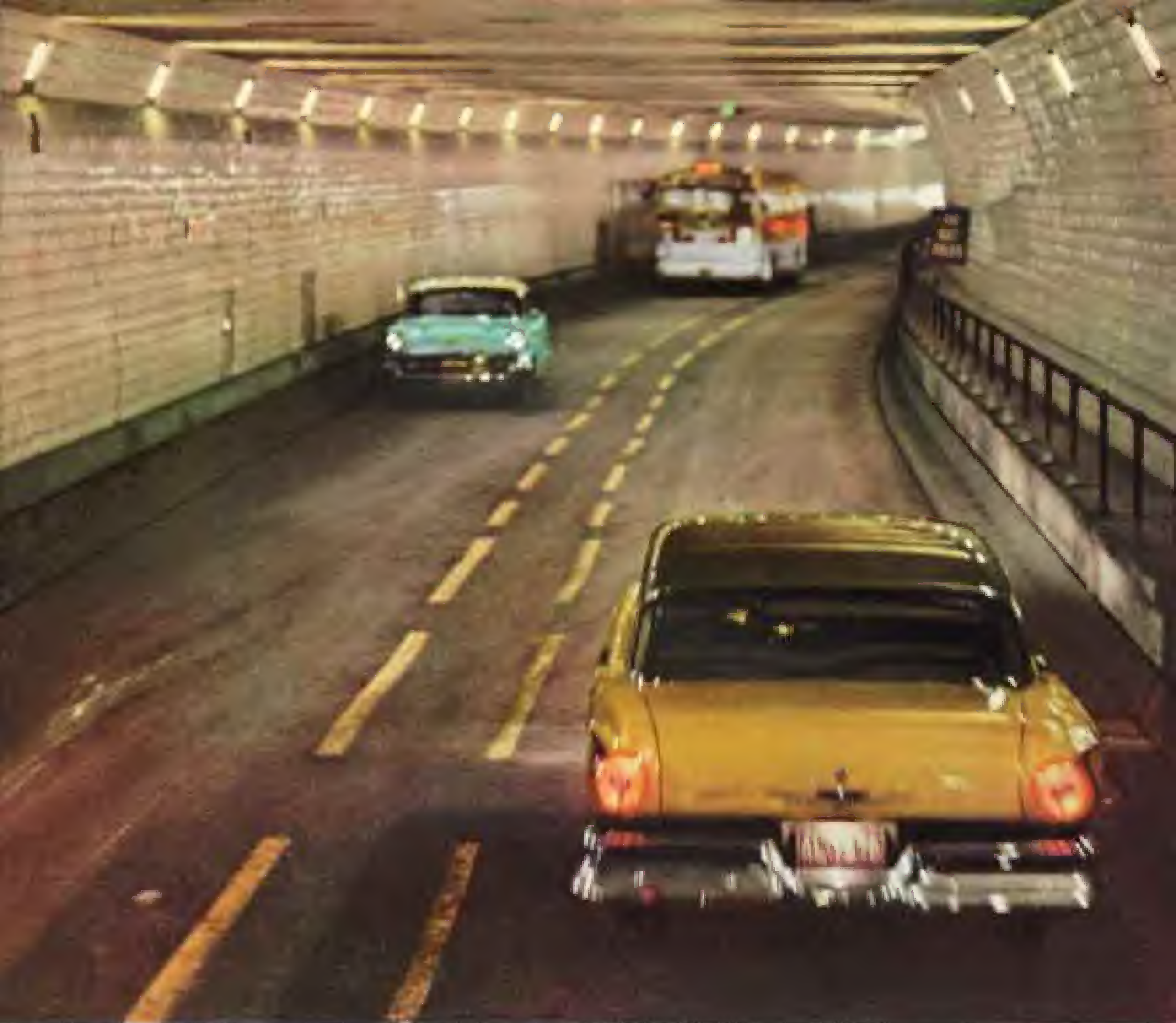
The Detroit-Windsor tunnel is one mile long—with 2300 feet of its length directly under the Detroit River.
