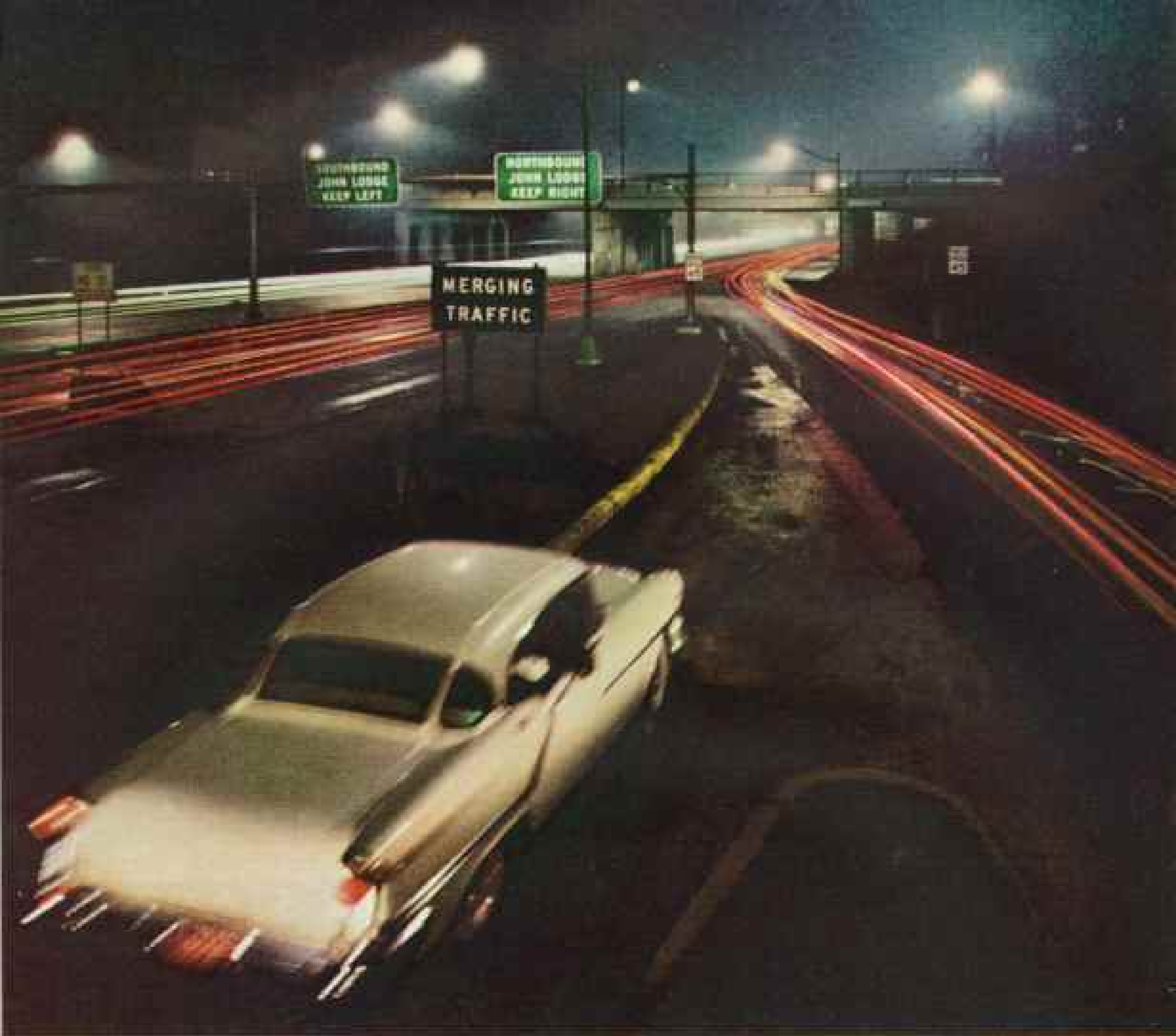
Approach ramp on Detroit, Michigan, expressway.
