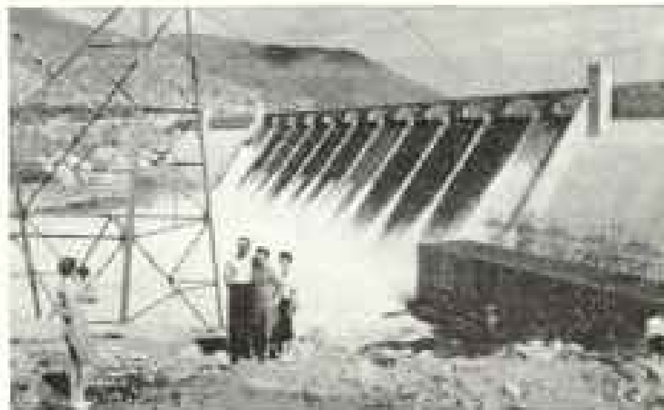
Grand Coulee Dam... almost a mile wide!
