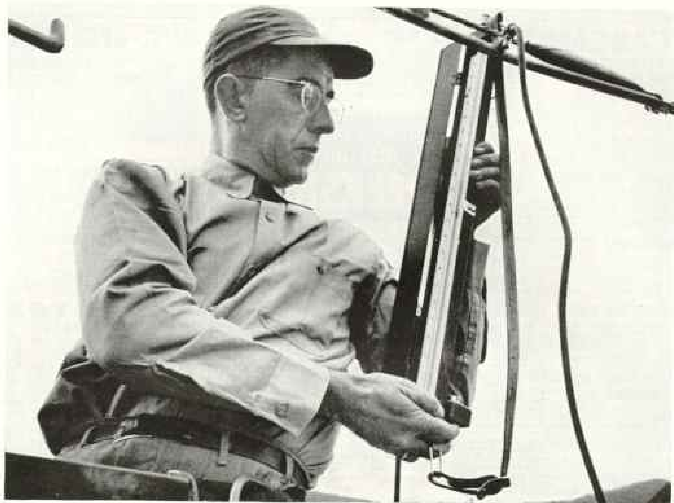
TELEPHONE MAN WORKING FOR YOU William T. Wright, Jr., regularly measures the pressure in telephone cables in order to help keep your telephone service trouble-free.
