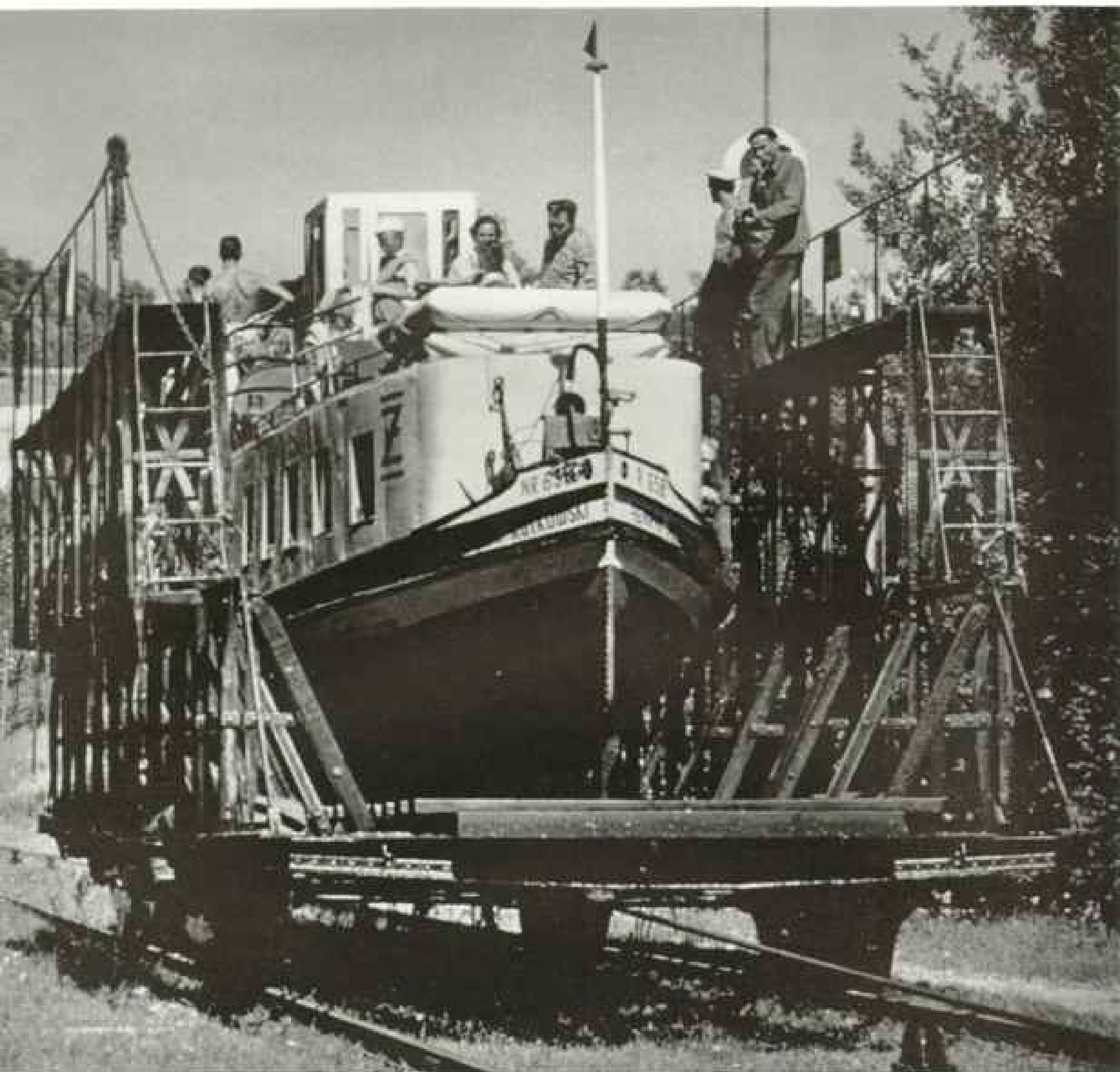
makes an over-the-hill portage on rails. Passengers enjoy a voyage past dense forest
