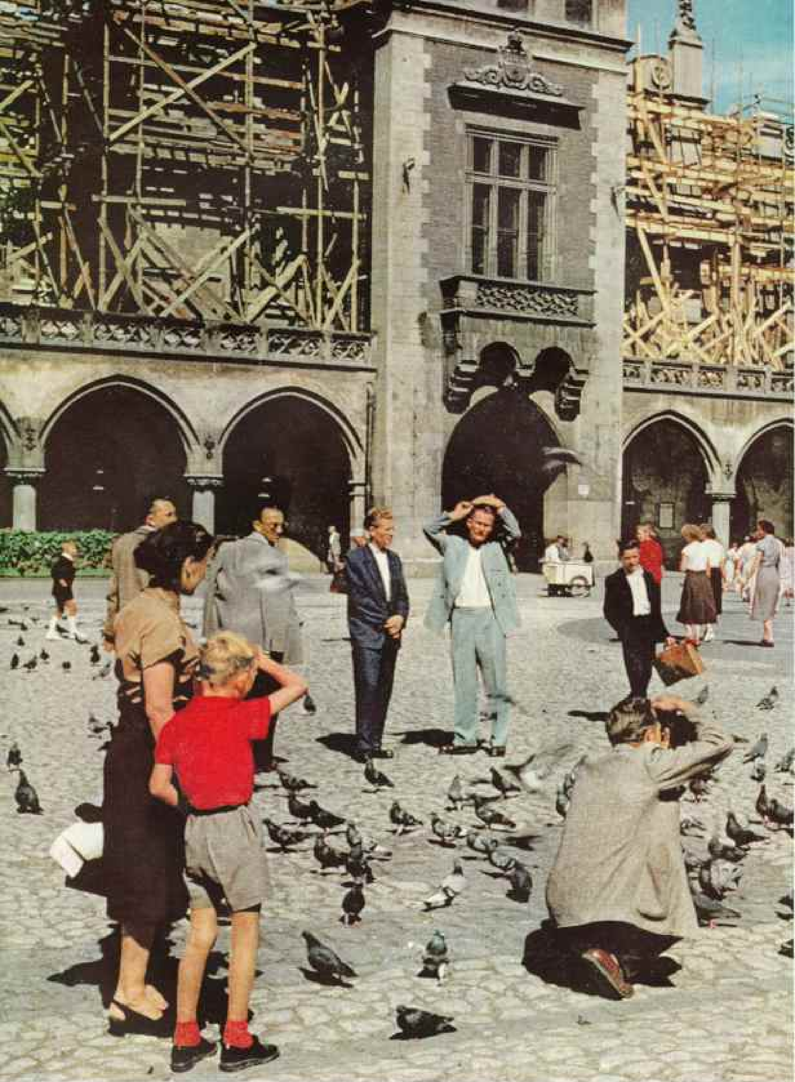
Kraków's Six-century-old Cloth Hall Wears the Scaffolding of Renovators
