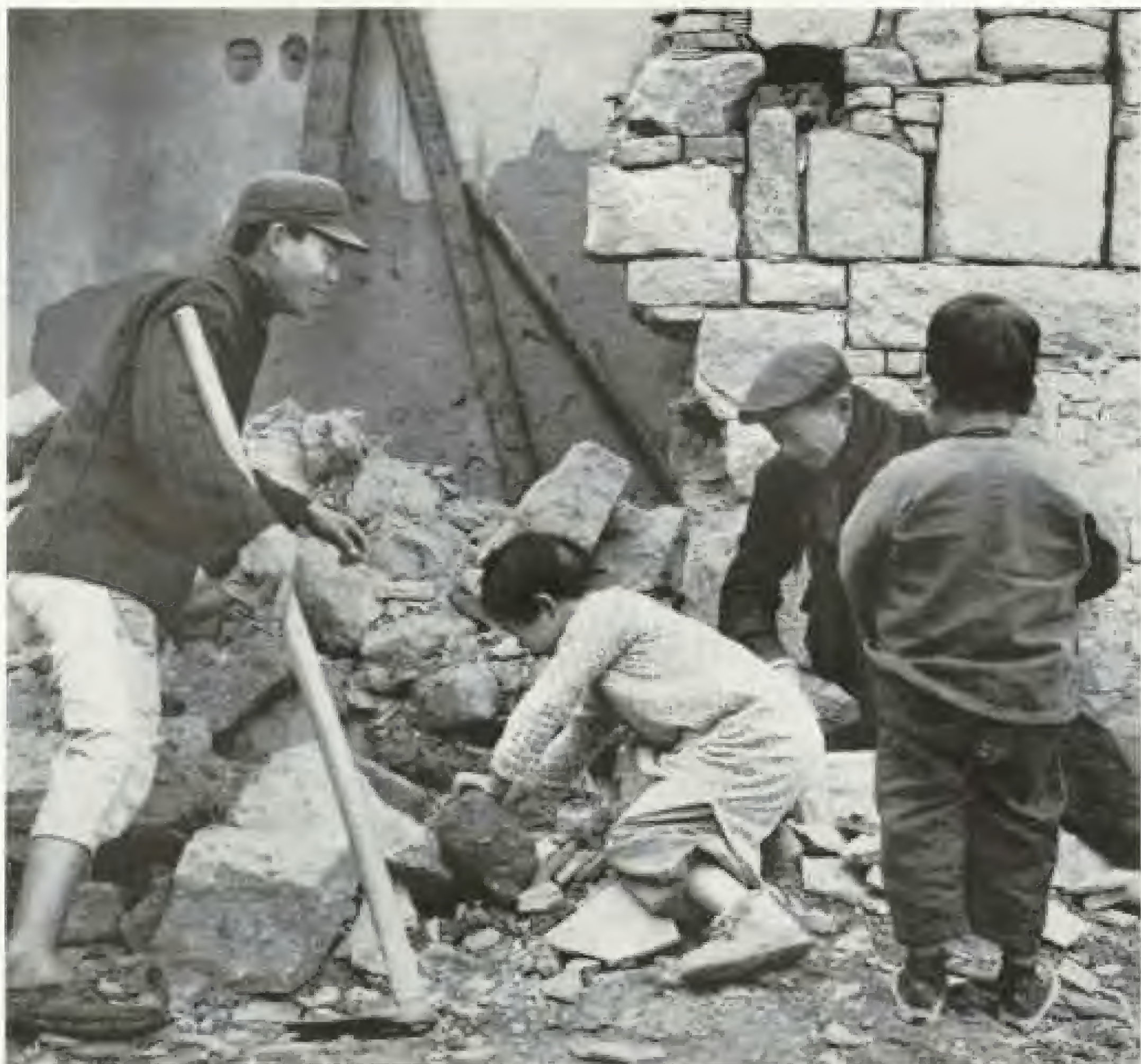
Salvage party searches rubble for belongings after a hit. Few houses stand unscathed. Barrages saturate the island, shattering hospitals, schools, and temples (opposite), as well as military targets. Dispossessed families live in caves (page 429).
