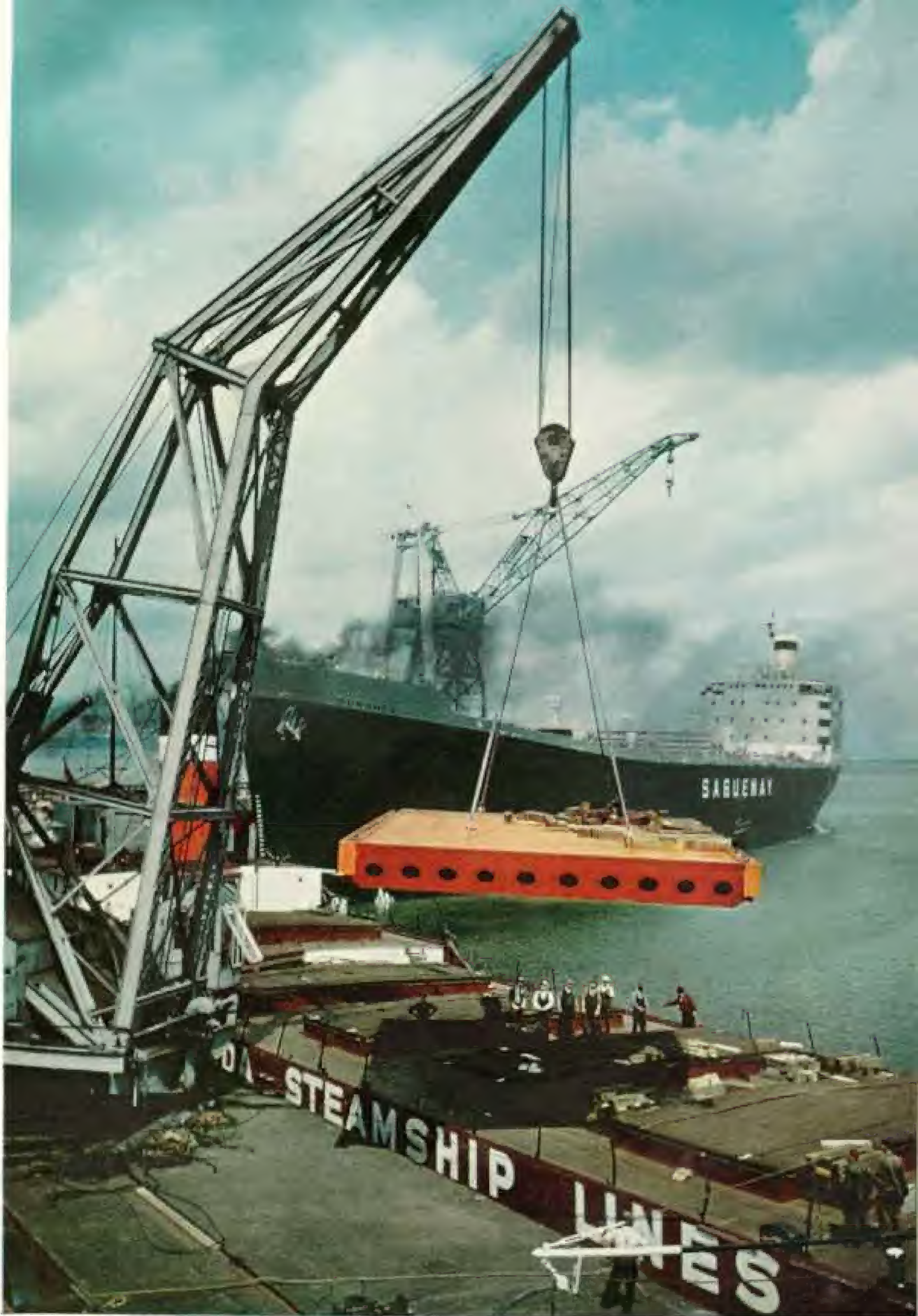
Gantry crane at Lauzon, Quebec, loads a 45-ton gate for the powerdam at Beauharnois. Newly launched, the Saguenay line's freighter Sunbeag carries an all-aluminum superstructure.
