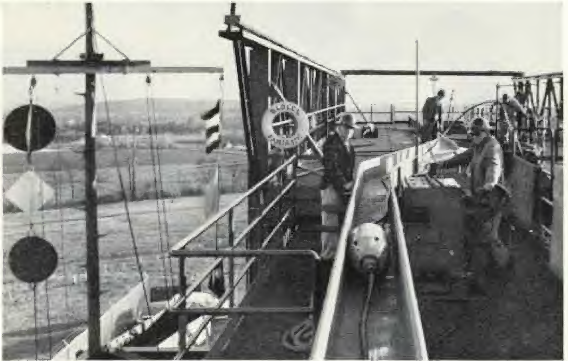
Engineers study section of cable containing dummy amplifier being payed out. Inscription on life preserver stands for "Bell Laboratories Dry Land Cable Ship Fantastic ."
