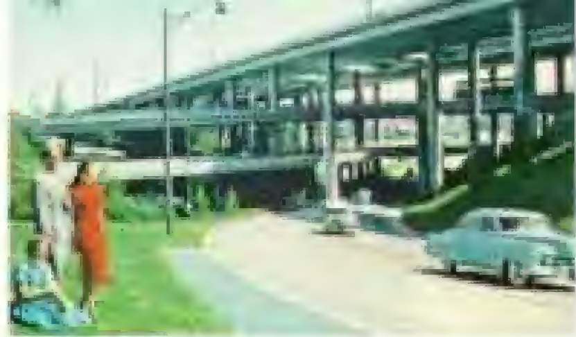
Drive our freeways to save time. This is the "Stack" downtown Los Angeles.
