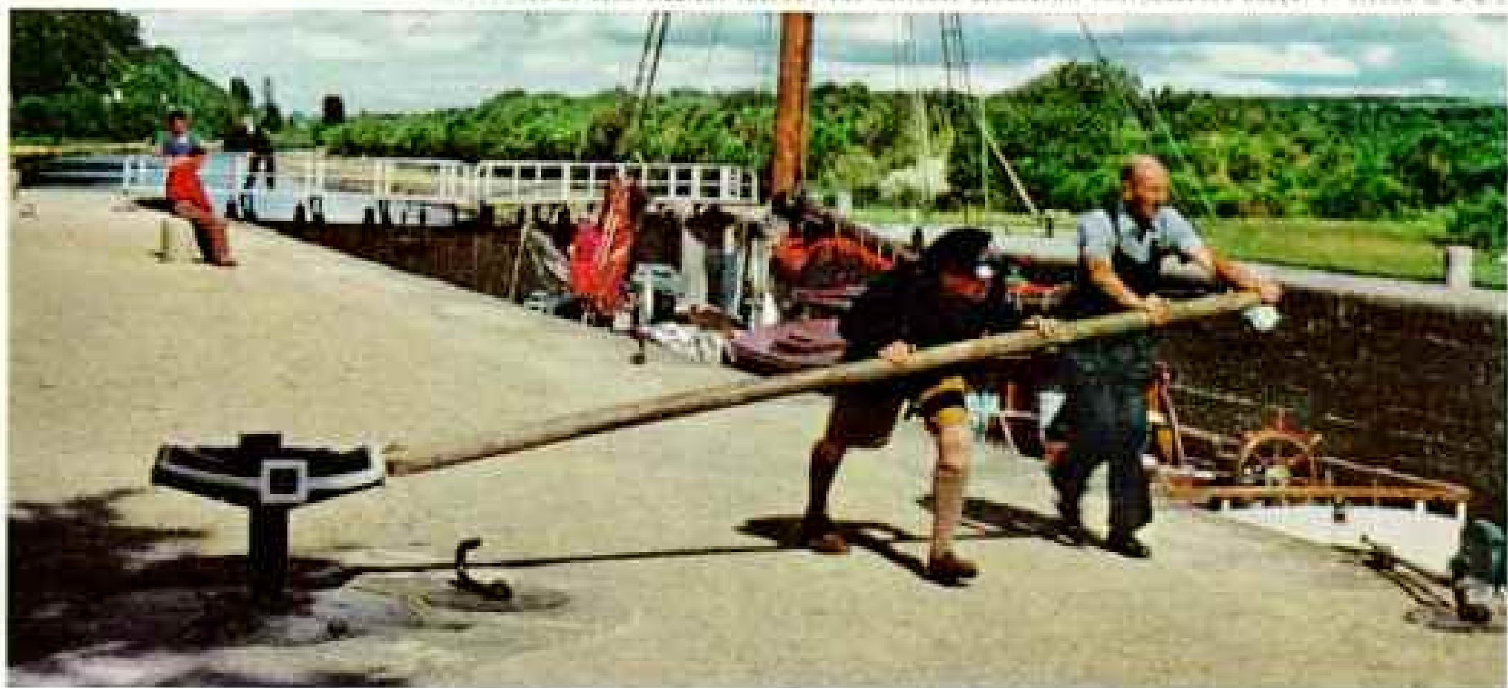
Heaves on a capstan bar swing lock gates on Scotland's Caledonian Canal. Cristoden's crew often helped keepers walk the gates open or shut.
