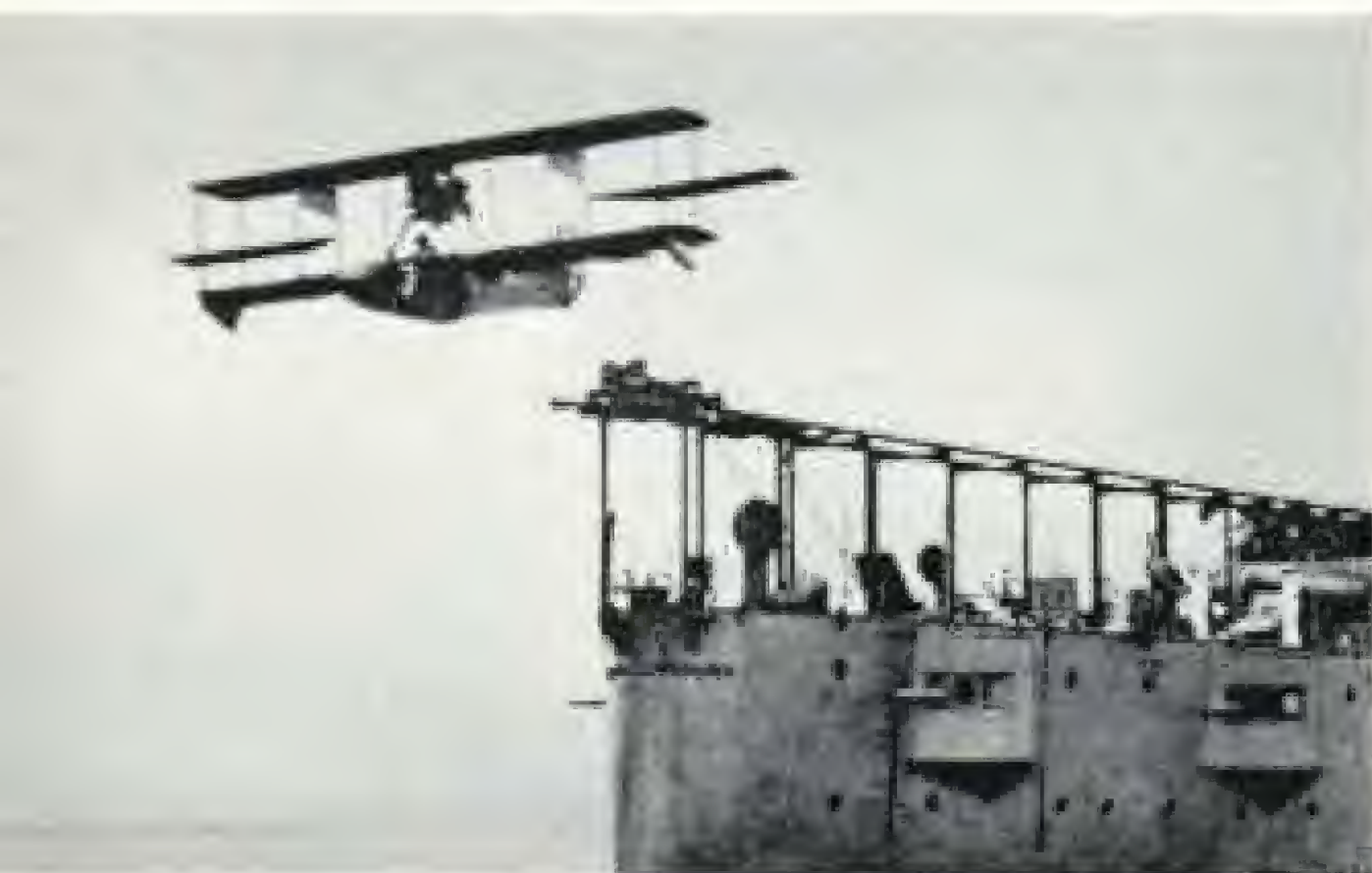
AB-3 Curtiss flying boat shoots from a permanent catapult installed on the stern of the U.S.S. North Carolina in 1916. The armored cruiser thus became the first naval ship equipped to carry and launch aircraft at sea.
