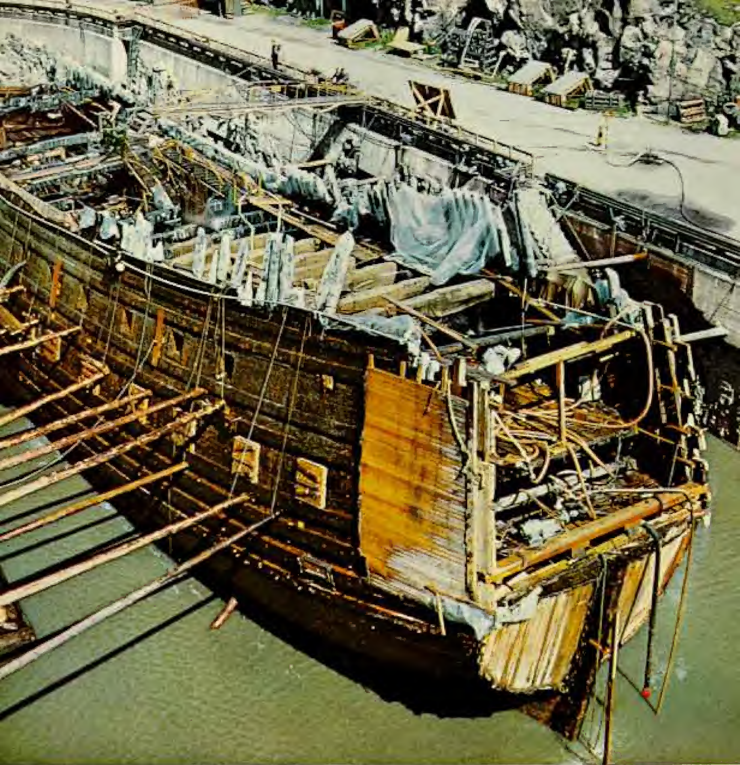
RECONSTRUCTED BY HANS LINDHOLM (ARROWS) AND W. E. RICHARDS, NATIONAL GEOGRAPHIC STAFF © N.G.S.
