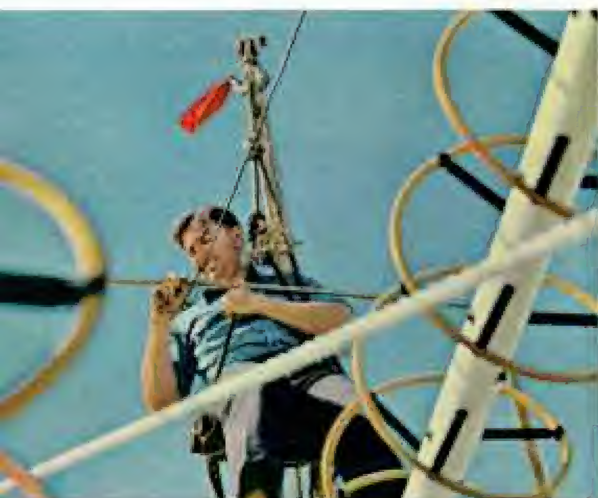
Block and tackle hoist an Aussie technician aloft to repair spiral antennas on a Muchea transmitter.
