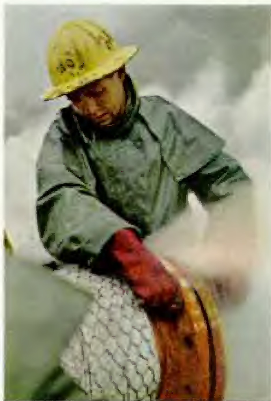
Scalding steam escapes from a pipe connection. Hard hat and rubber coat and gloves protect the workman.
