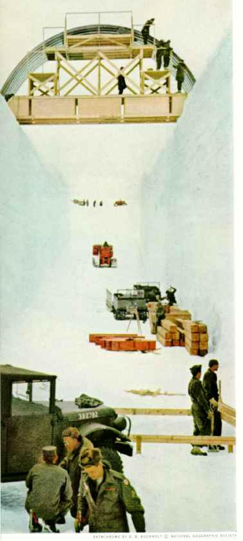
Atomic reactor trench takes shape at Camp Century, 886 miles from the North Pole. United States Army Engineers, who installed the nuclear plant, worked 12- to 14-hour shifts and used some six thousand tons of supplies and equipment.
