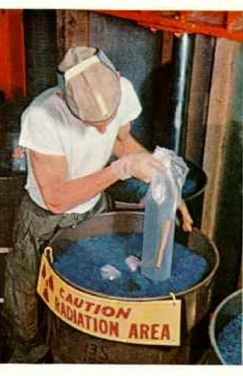
Unpacking atomic fuel, a technician wears rubber gloves to keep these elements clean after removal of plastic wrapping. Forty-three pounds of uranium will operate Century's atomic plant for two years.
