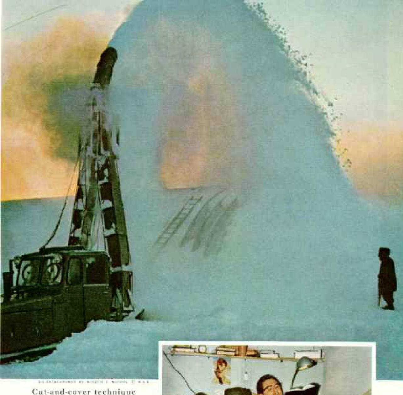
Cut-and-cover technique stemmed from several years of experiments in Greenland. Powerful Swiss plows called Peter Snow Millers cut trenches as deep as 35 feet and hundreds of feet long. Men roof the trenches with overlapping steel arches and spray snow onto the roof, where it solidifies.
