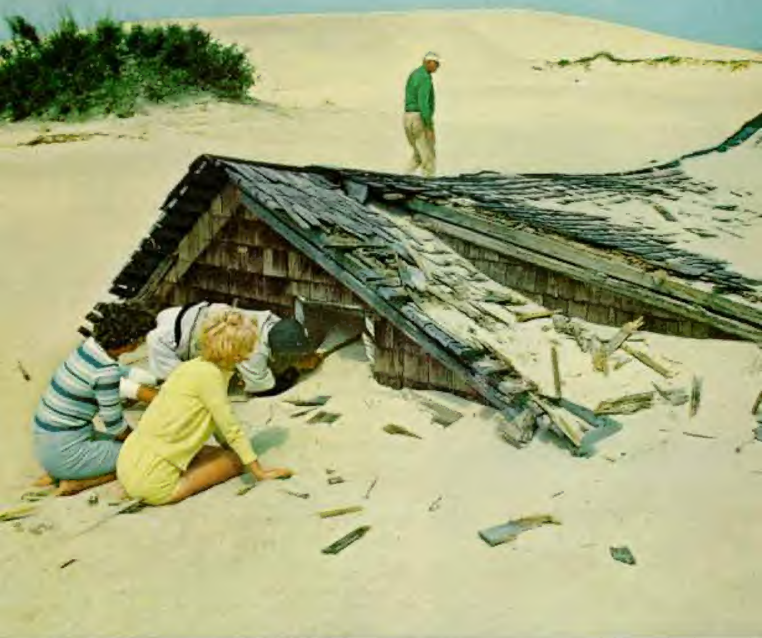
Buried to the eaves, this beachside house once sheltered a fisherman's family. Creeping inland, the sea of sand engulfed the village of Wash Woods, North Carolina.
