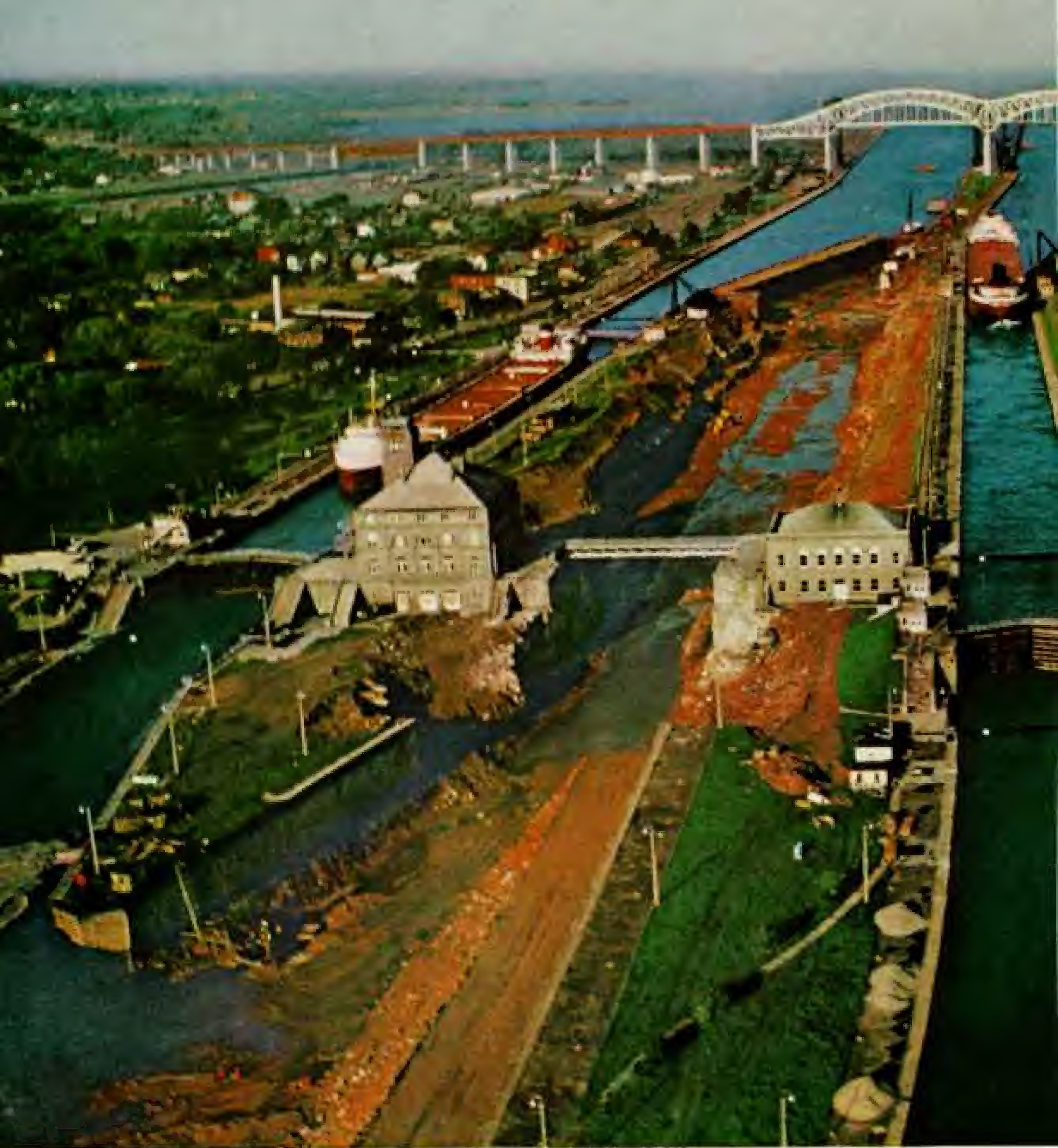
Sault Ste. Marie Locks, in the busy Soo Canal, lift Great Lakes carriers over a 22-foot drop
