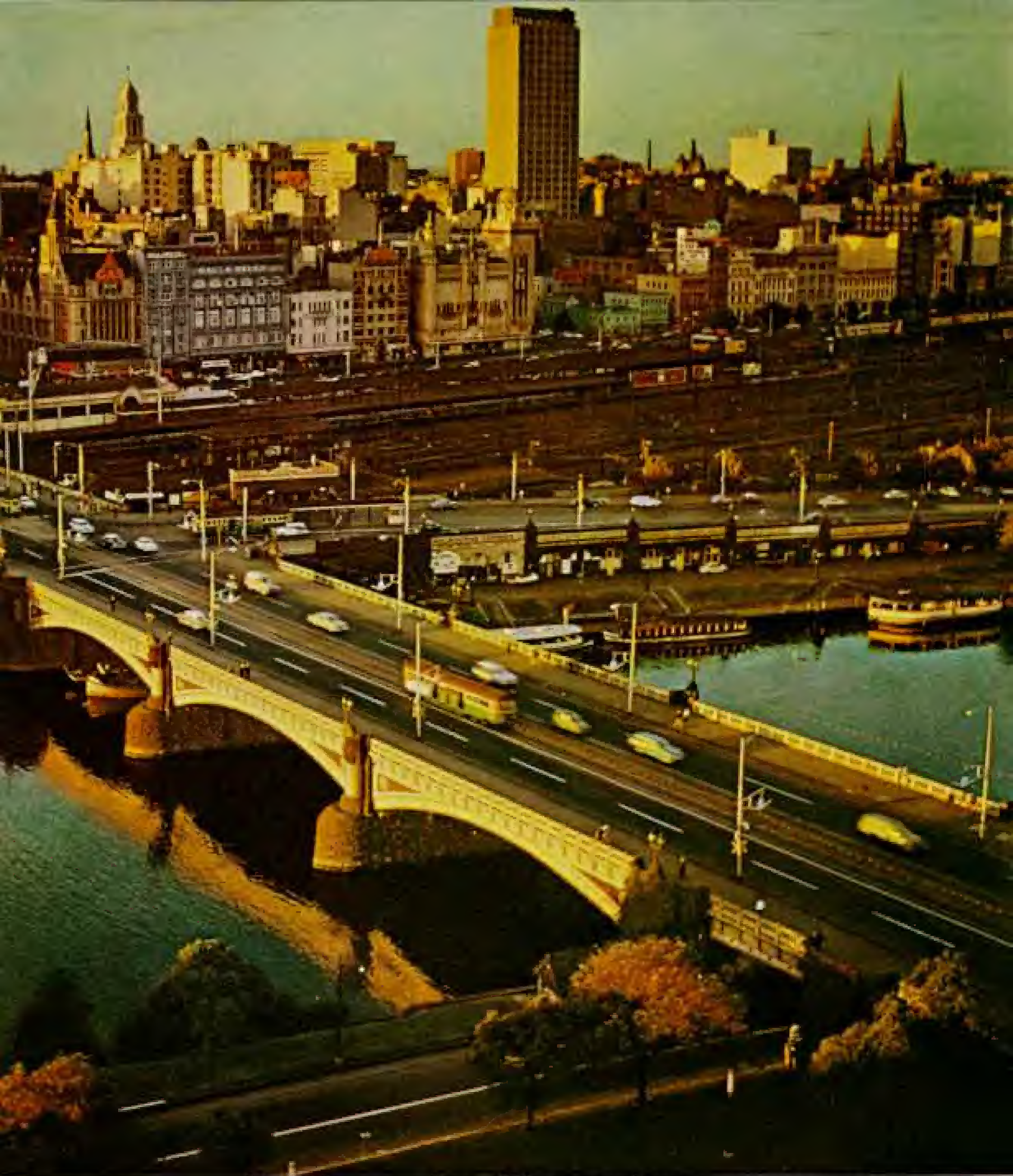
PHOTOGRAPH BY GORDON IN JULY 1963. THE BRIDGE-TYPE BY GILBERT C. JOHNSON. © W.R.C.
