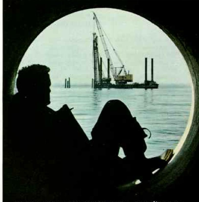
UNIQUE BIG D HOPS ACROSS THE SEA, pounding concrete piles into the bay's sandy floor. Hollow pile above,  $4\frac{1}{2}$  feet in diameter, shelters a worker. Diagram shows the \$1,500,000 rig standing on the bottom as it drives piles in sets of three. Tubes go as deep as 100 feet, where sediment and friction hold them fast. Lifting its legs, the massive hammer then floats to a new position.
