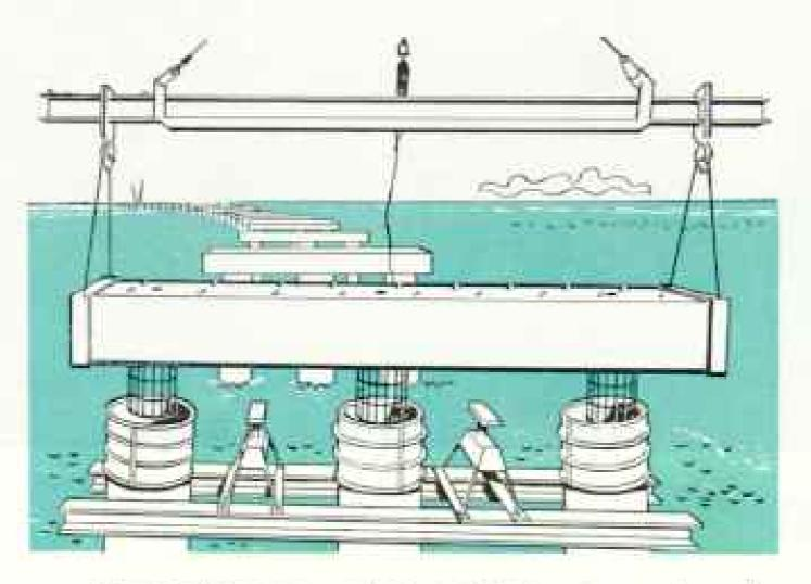
Twenty-ton cap, ready for installation, bovers above the trimmed piles. Plugs of latticed steel to reinforce concrete will fit precisely into pile tops.
