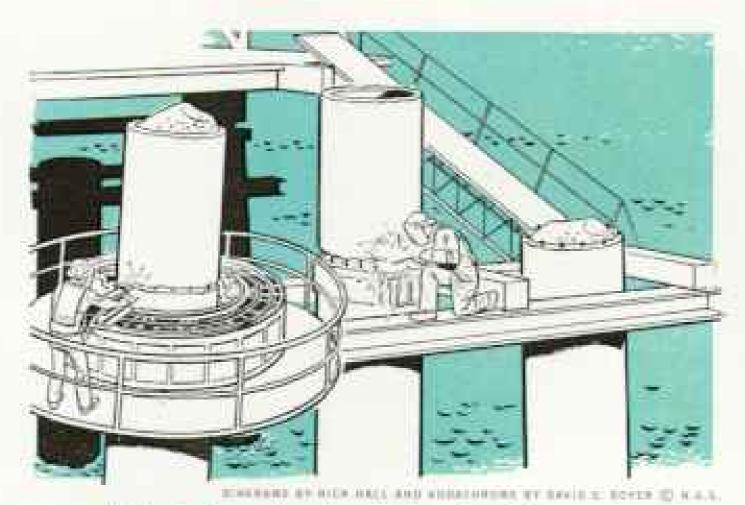
Helmeted workers level the piles. Man at left, guiding a jackhammer on a circular track, chips through a five-inch wall of concrete. Acetylene torch of worker in center cuts wires that are bunched together as in a cable and threaded through 16 holes in the tube's lining.
