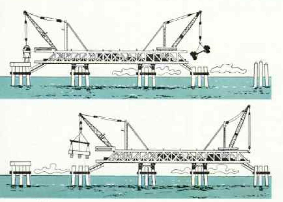
Two-headed Monster, as engineers call it, skates on piles that will support the roadbed. Machine's right end levels the piles by cutting them off or building them up. Left end caps three sand-loaded tubes.
