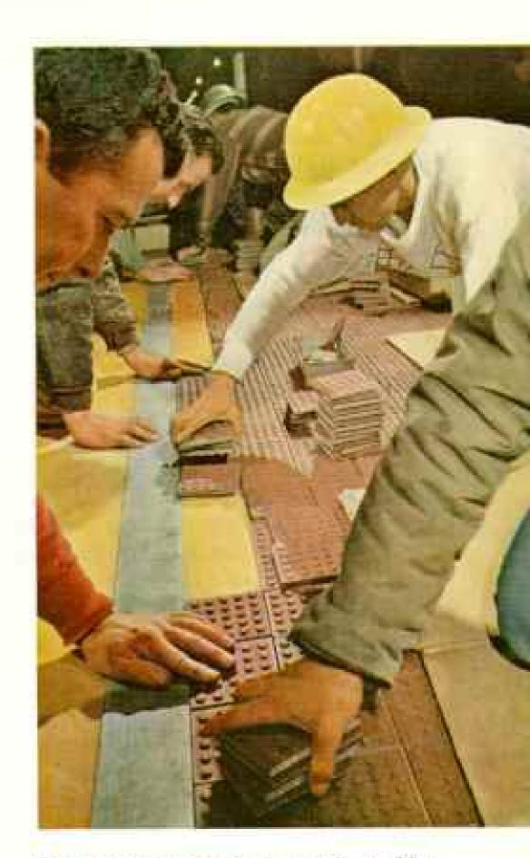
Reverse twist on the tilesetter's art: Men working on a platform beneath the tunnel's arched ceiling (left) lay rows of tiles face down on a dry form. Concrete is then poured over the bottoms of the tiles to make a false ceiling (below) for air ducts. Height of the two-lane tunnel; 14 feet.
