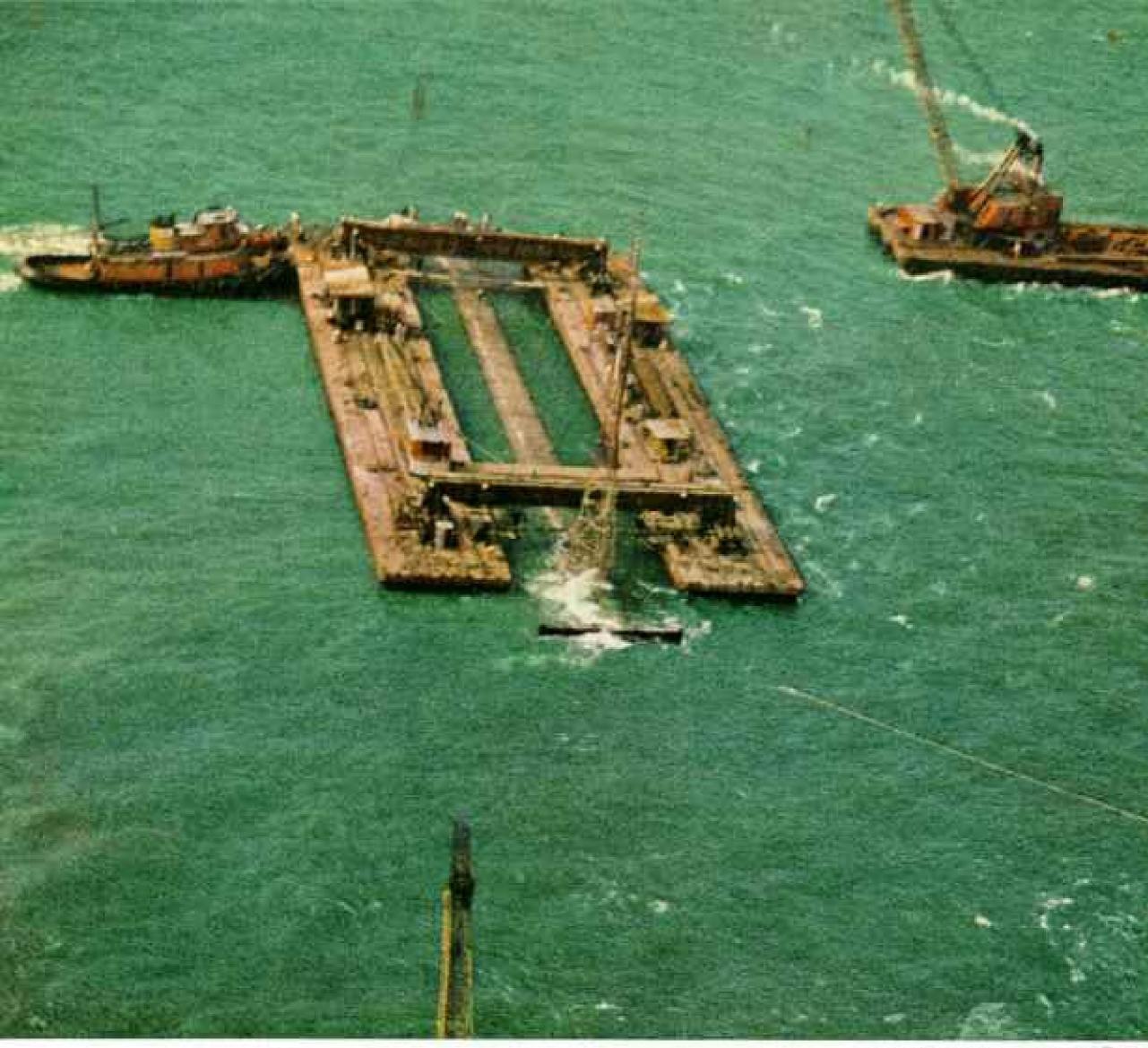
Twin Barges Hold a 287-foot Tunnel Section as Tugs Pull and Push the Assembly to Sea
