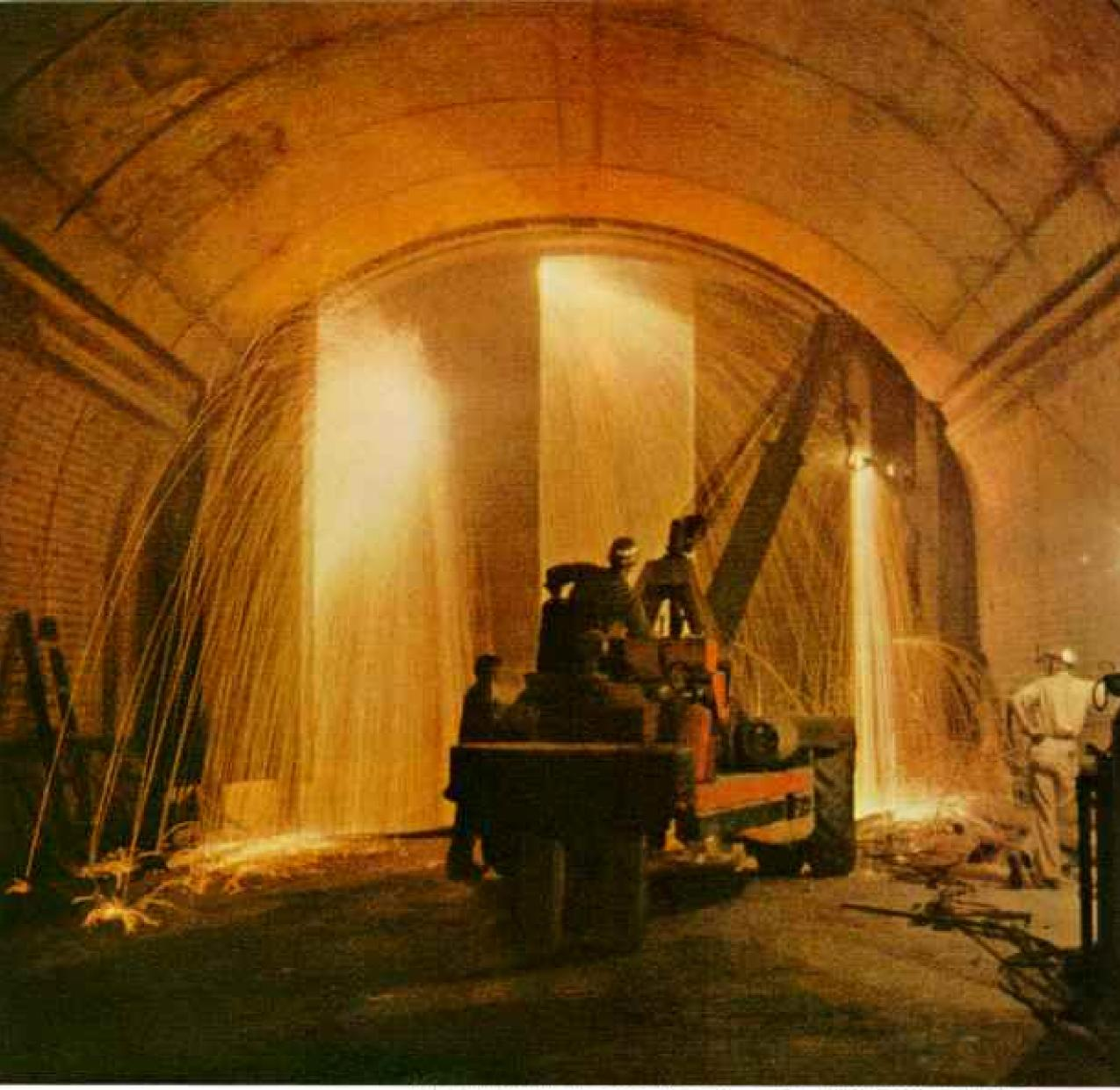
Sparks fly as welders cut away a steel bulkhead separating two sections of tunnel.
