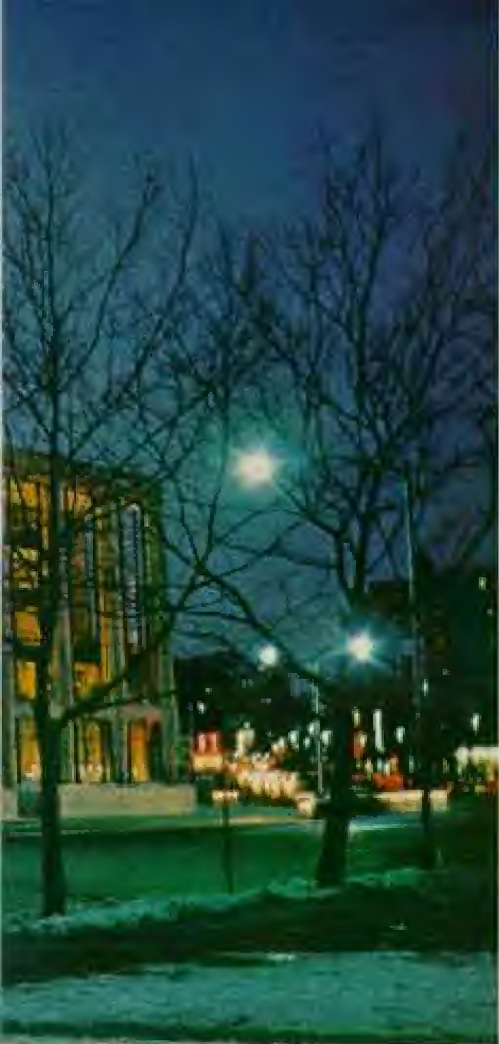
a library-museum; and the Juilliard School of Music. The $160,700,000 project is due for completion in 1967.
