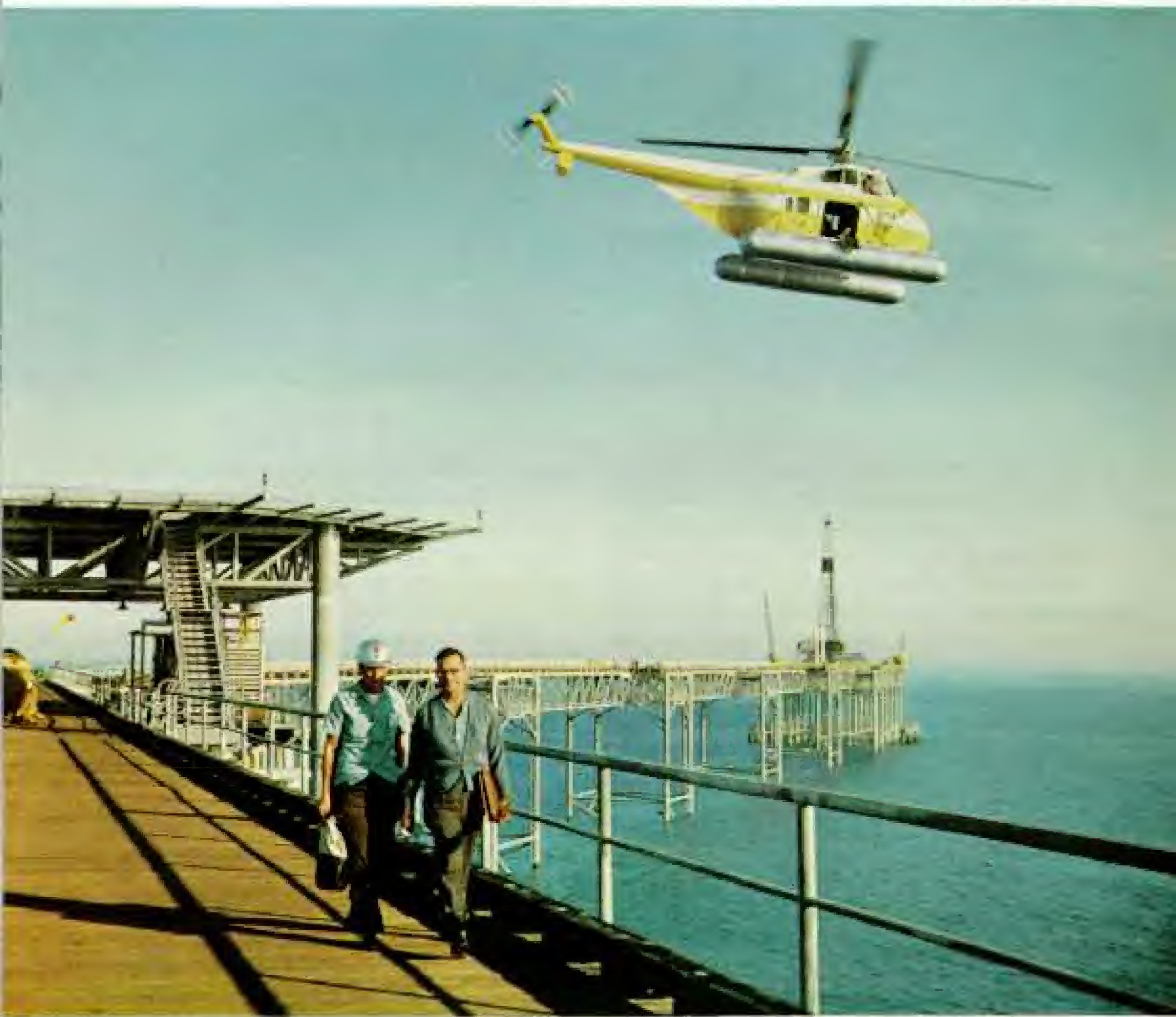
Blades whirring, a helicopter chugs aloft from Freeport Sulphur's mile-long Y-shaped mining platform off the Louisiana coast. Here superheated water, forced 2,000 feet beneath the Gulf to a subterranean deposit, melts the sulphur. Conveyed by pipeline to shore, 80 percent of the mineral goes into storage for sale in liquid form; the remainder solidifies in vats at Port Sulphur (opposite).
