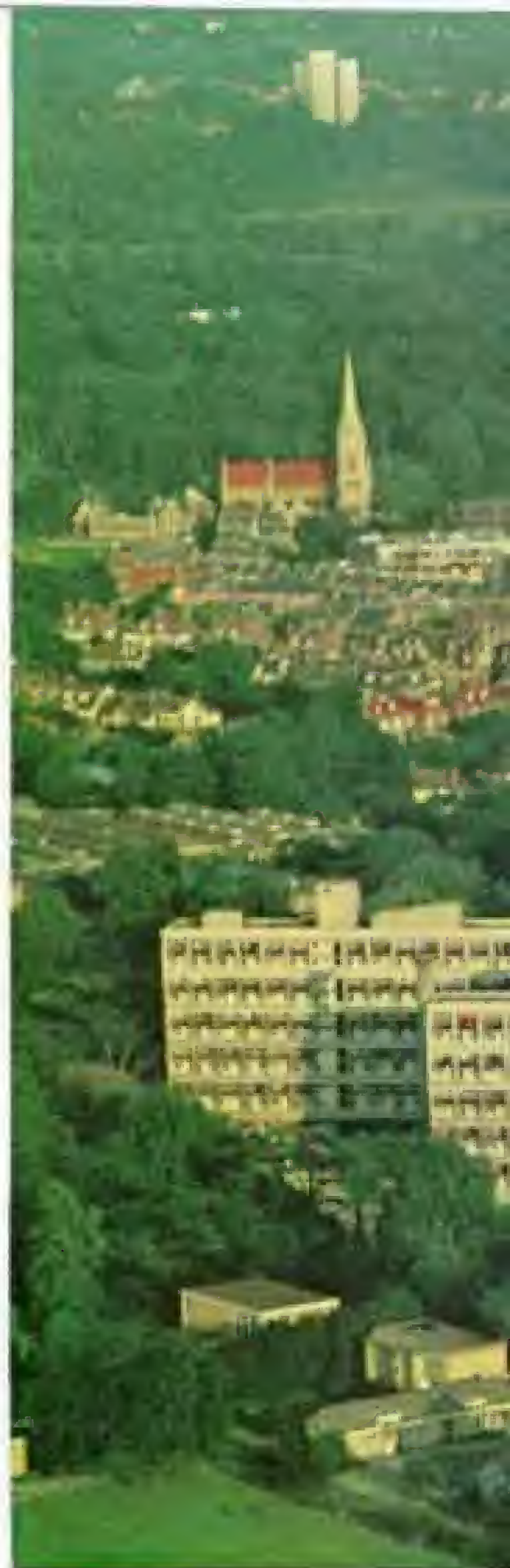
Homes for thousands , high-rise apartments of Alton East and Alton West lift above the village of Roehampton and its spired church. Six miles from the heart of London, the development houses low-income families. One-story bungalows scattered through the parklike grounds provide accommodations for the elderly.
