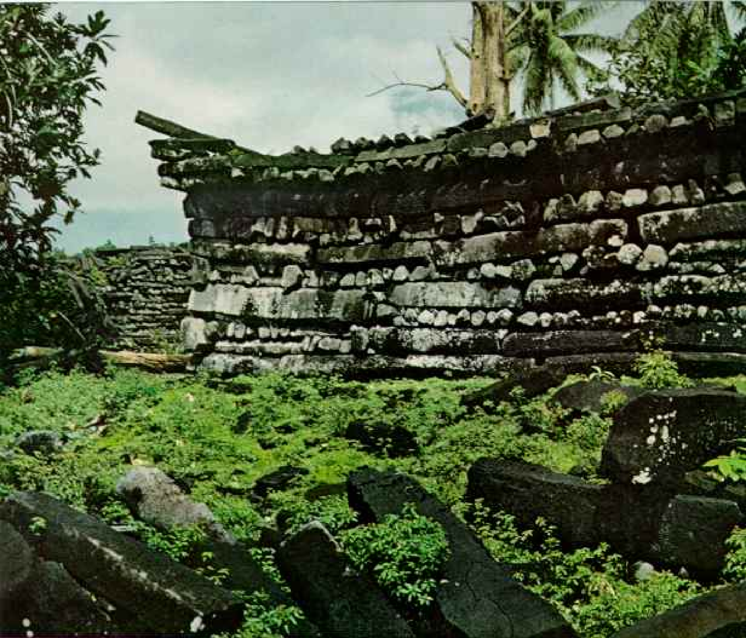
Haunting ruins of Nanmatol pose a riddle for archeologists. Built on Ponape of rock "logs"—huge crystals of basalt found on the island—such enclosures spread over a hundred islets that fill a swampy lagoon. Local legend hints that the structures' owners were tyrants who
