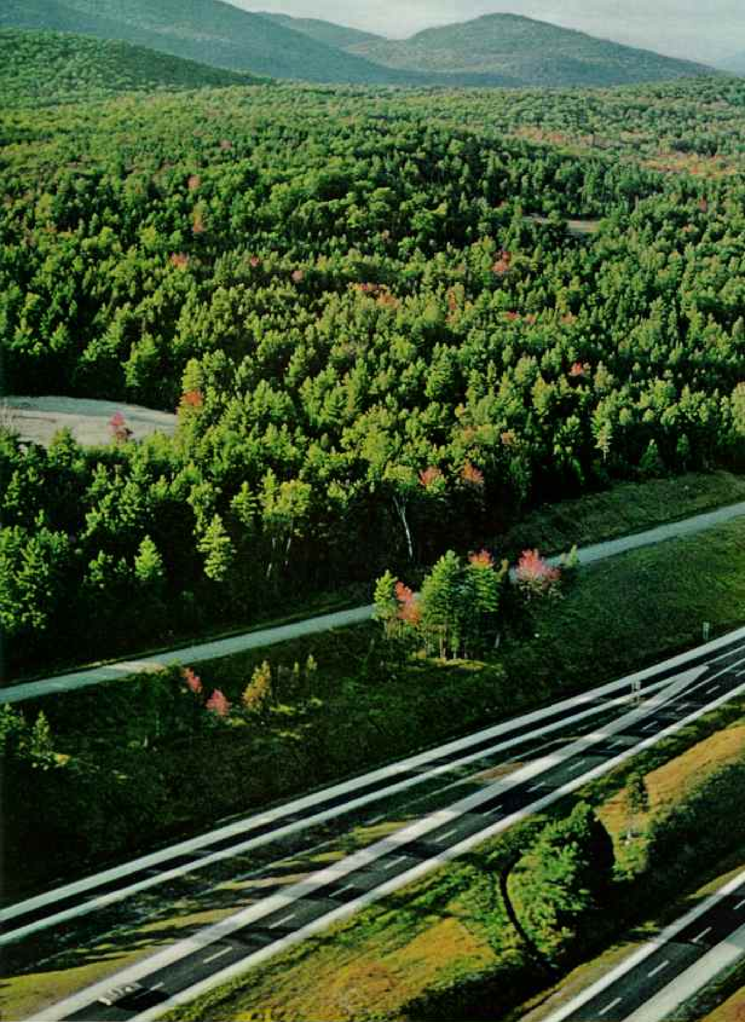
Highroad to the wild green yonder, New York's Northway sweeps majestically through the Adirondacks. Planning for safety and beauty, engineers walked every step of the route from Albany to the Canadian border. Their dreams fashioned a highway for the future with parklike dividers
