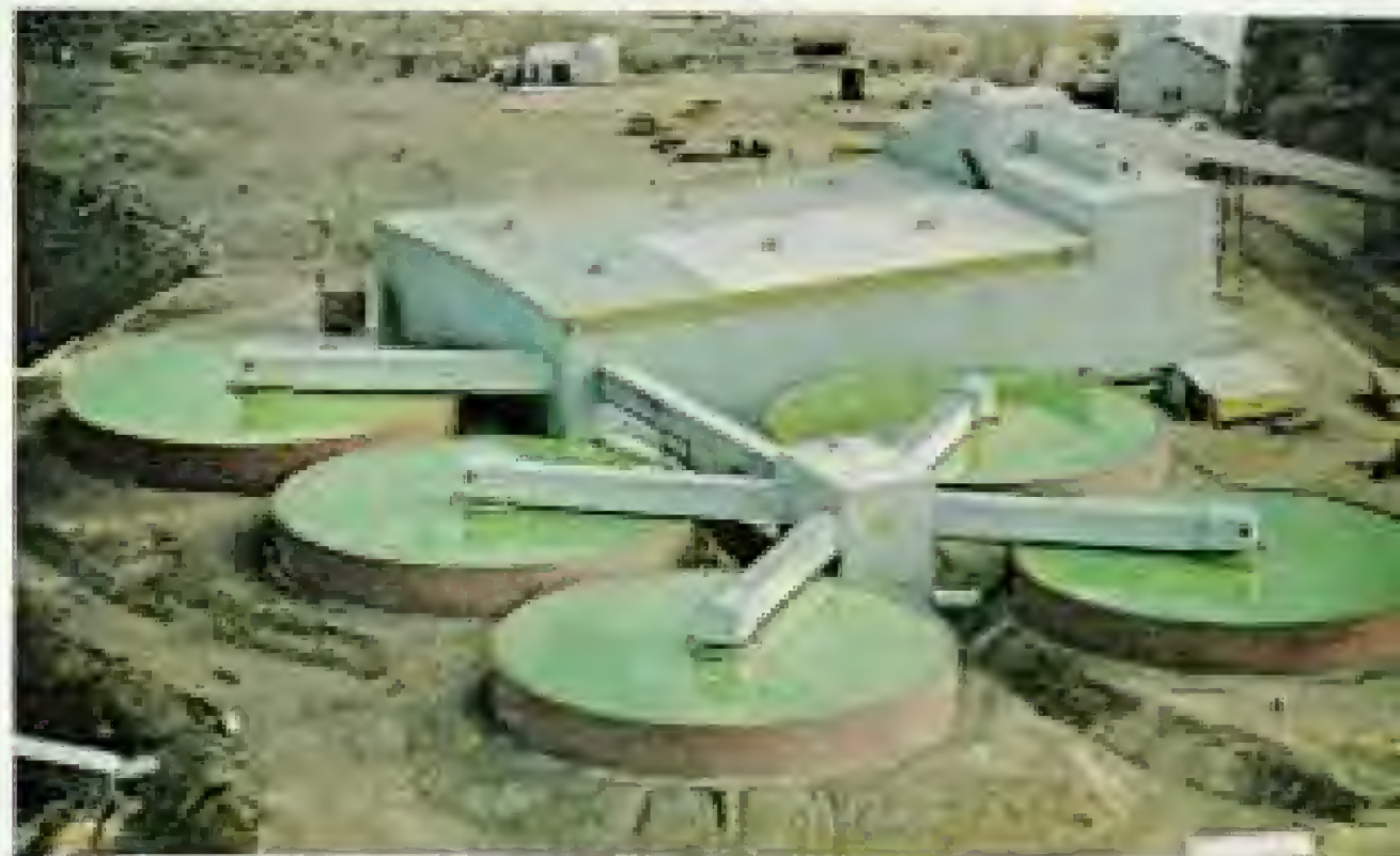
Thickener tanks settle out waste while gold-bearing cyanide, called pregnant solution, flows off the top.
