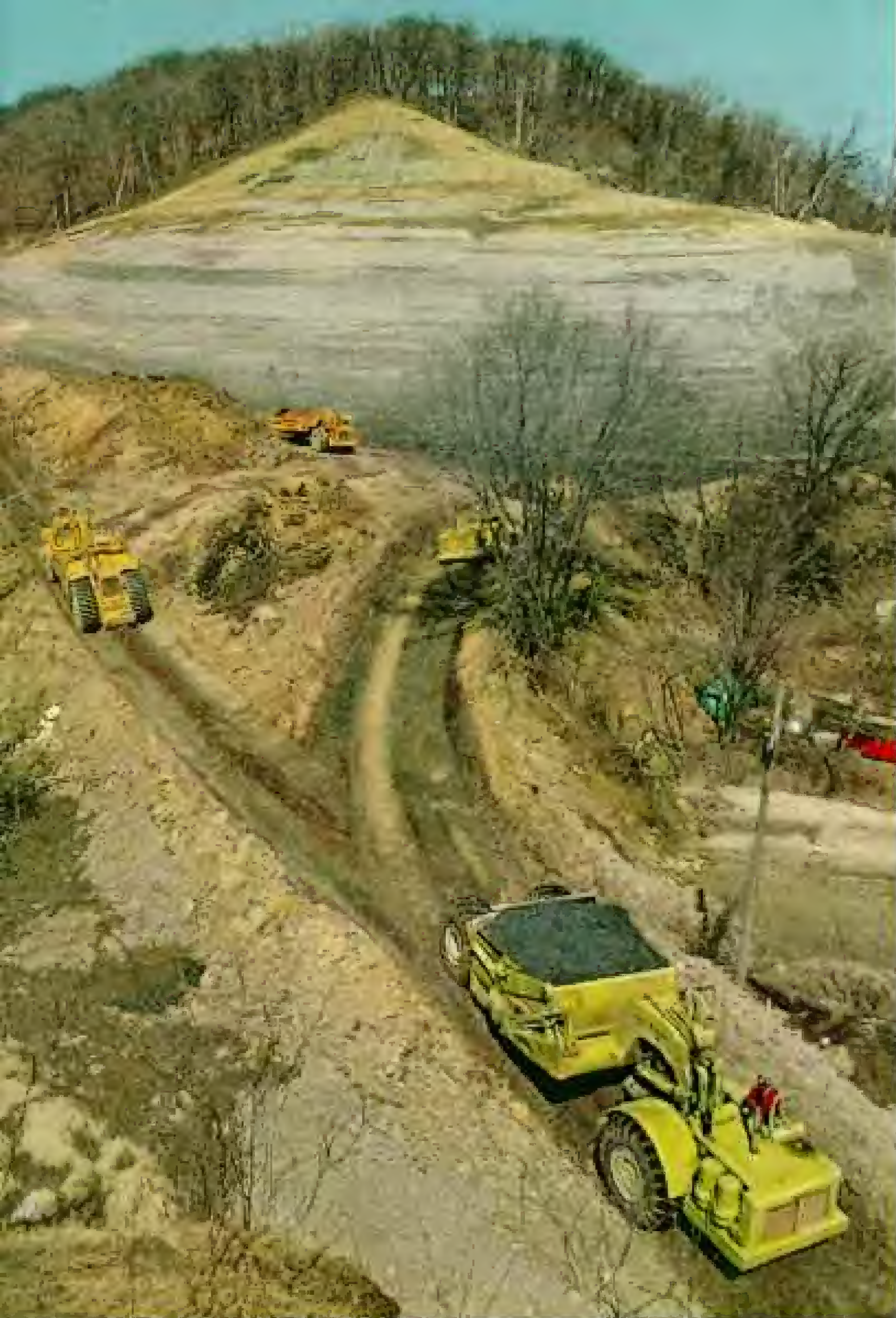
Moving a hillside to tame a river: Hungry scrapers gulp huge loads of earth to build up a North Mankato dike. The region's rich blue-gray clay proved ideal for making watertight levees.
