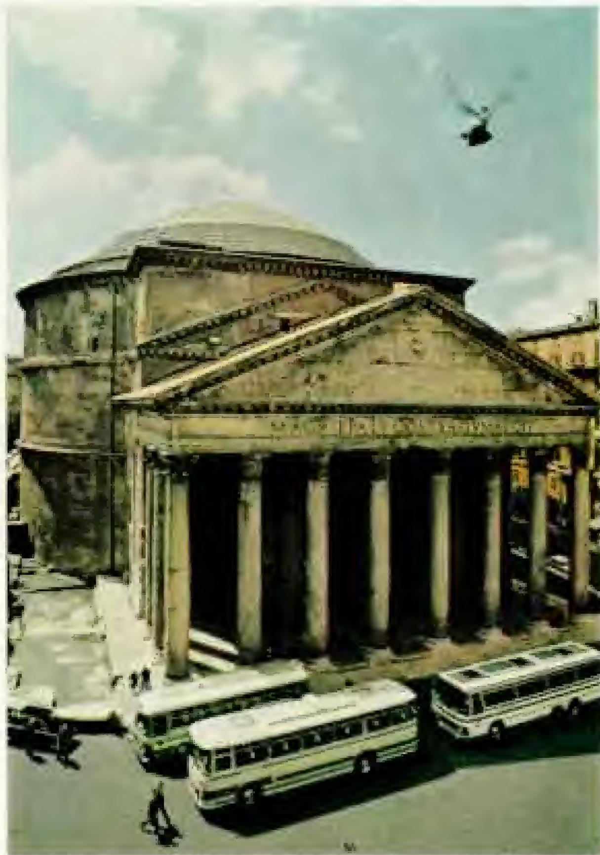
EXTERIOR (LEFT) AND INTERIOR OF ROMAN PANTEON © N. G. P.
