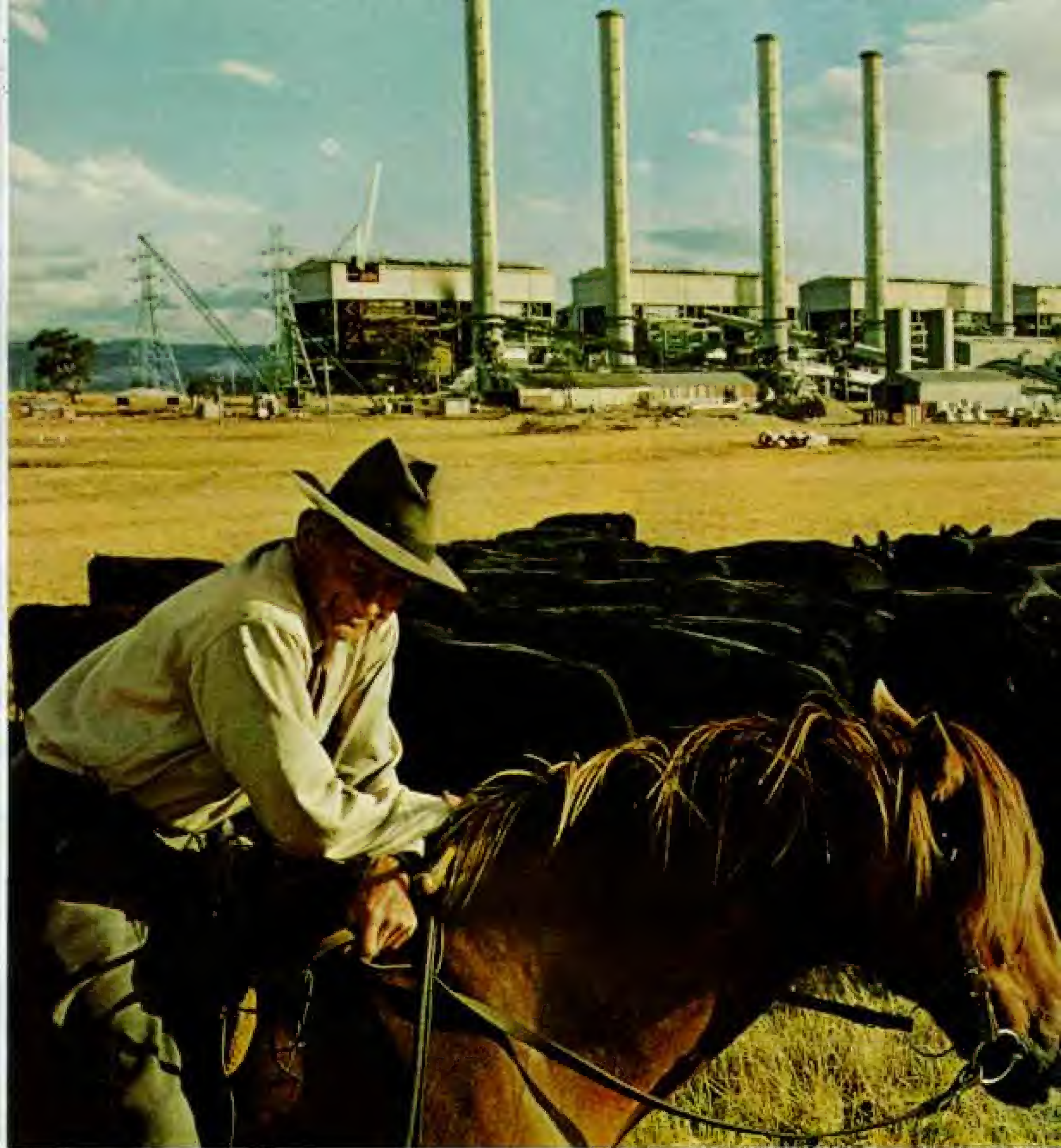
New neighbor on the old range: The coal-burning Hazelwood Power Station rises on pastureland near Morwell, previously owned by Alfred Ronald, who retains grazing rights for his Aberdeen Angus herd. Facing displacement, the nearby town of Yallourn, built
