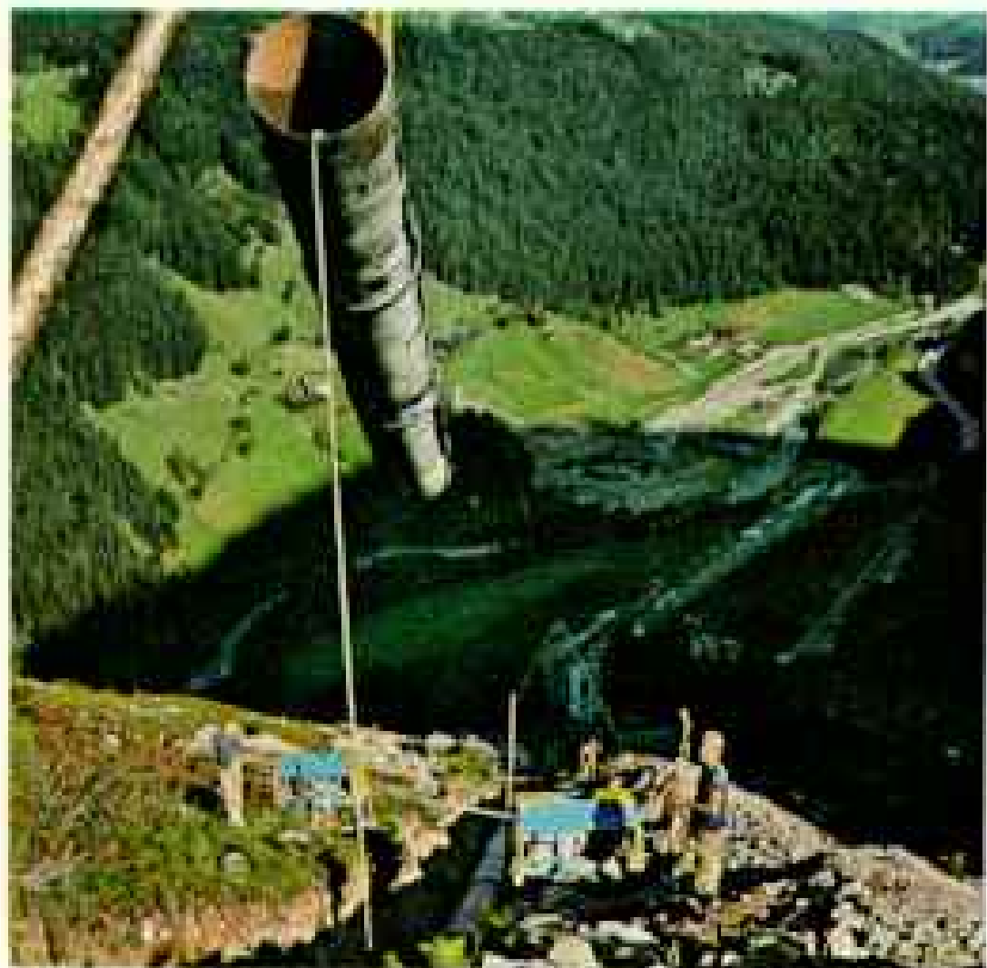
In rocky terrain, the pipe is laid on a cushion of sand to protect it from jagged projections.
