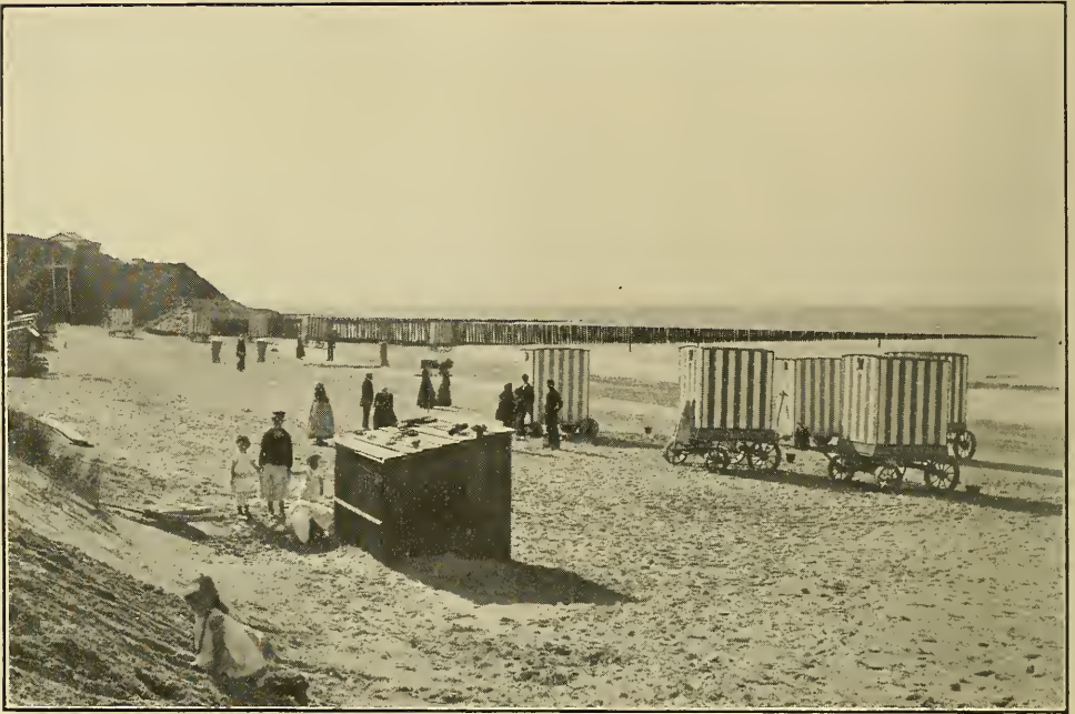
Pile Dikes for Protection against Marine Erosion
