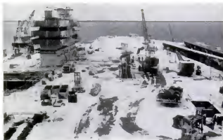
SNOW COVERS "FORRESTAL'S" DECK AS CONSTRUCTION GOES ON
