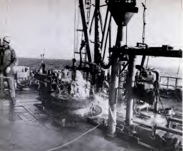
(RIGHT) SQUIRTS UP PIPE. DIALS MEASURE PIPE'S WEIGHT AND TORQUE
