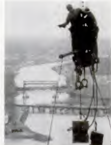
RIDING THE HOIST , two bridgemen are swung by the derrick from one side of bridge to another, 60 feet away. This is unsafe, frowned on by company.
