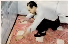
INSTALL IT YOURSELF! Sandran has flat without leveling—or cement if you prefer. Just cut to shape and roll in place. Comes in rolls 6 and 9 feet wide to fit room size rugs.
