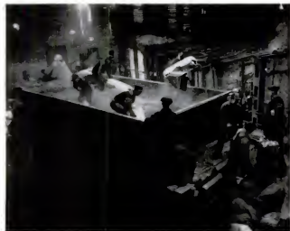
IN THE FREIGHT CAR the ingot is quickly covered with vermiculite. The insulating characteristics of the mineral are so effective that the workmen can walk around on the red-hot ingot as soon as it has a two-inch covering. Dominion gets its vermiculite from the Zonolite Co.'s mines in Libby, Mont.
