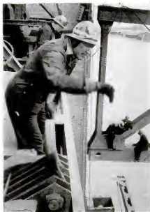
"PUSHER," or foreman, Ben Roberts heads the raising gang which lifts steel from the barges below and fastens it temporarily in place for riveting gang.
