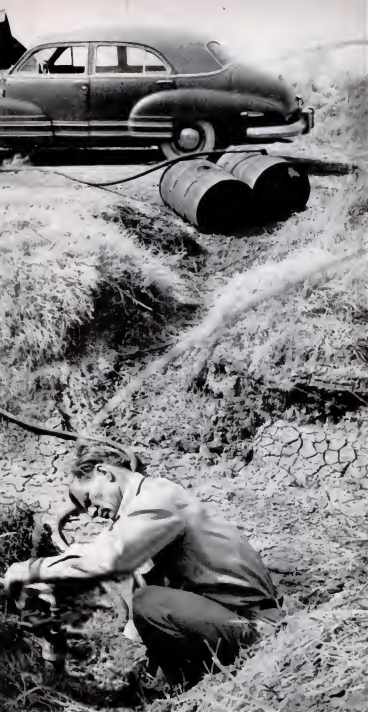
tank in rear, which is made from an old hot-water heater. Suction comes from vacuum pump which operates car's windshield wiper. Later oil is piped off into drums. Ratliff, in background, is checking oil flow through a window in the pipe.
