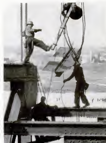
GUIDING A PLATE into place, bridgeman hangs on suspender with one hand and gives the tackle a kick with his foot. In the background is New Jersey.
