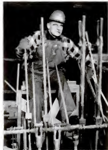
HOISTING ENGINEER York Smith runs a derrick on the tower, lifts loads he often cannot see. One false move by him could knock whole crew off bridge.
