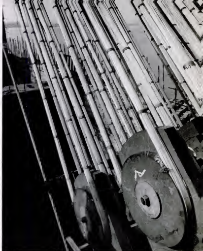
CABLE ANCHORAGE holds main cable at ends of bridge. Main cable is made of 19 smaller strands, each of which has 436 wires. All are looped around "hoop," which is in turn anchored in the masonry. Anchorage will be encased in concrete.
