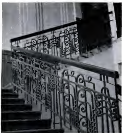
FIRST COMMISSION as a journeyman was to build this intricate wrought-iron banister for district court of Sisak.
