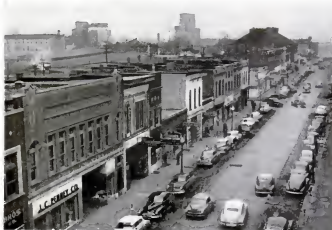
MAIN STREET RUNS TO RIVER ON WHOSE BANKS STAND GRAIN ELEVATORS
