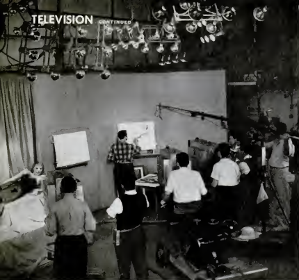
IN STUDIO during the broadcast of an art class, one camera covers the artist (center), another his model. A third prepares to shoot a new angle. The images are transmitted to control room.
