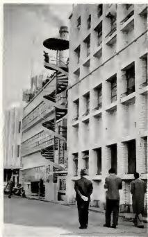
EXTERIOR IS FANCY, with a broad expanse of windows and spiral staircase down from roof garden.
