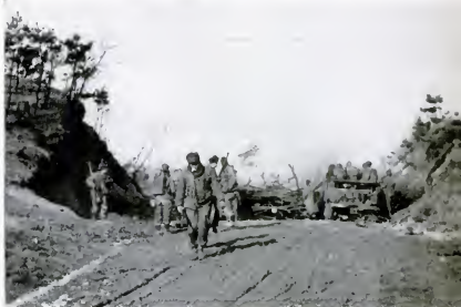
HALF-TRACK CANNOT PUSH THROUGH AND PLATOON BEGINS TO WITHDRAW
