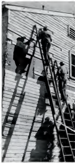
ROTTEN SIDEBORDS are torn off and replaced with new lumber.
