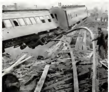
HANGING IN AIR, one of The Broker's cars juts out across overpass. Temporary trestle is at right.
