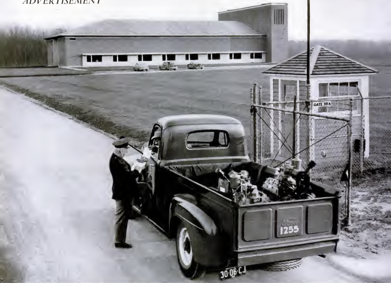
BEHIND GUARDED GATES lies the most advanced engine research center in the world—the new Ford Engine Test Laboratory. Completed in June 1949, this first wing of the Dynamometer Building houses fourteen dynamometers—intricate testing devices capable of duplicating any possible driving conditions and then
