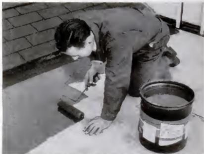
**CONSTRUCTING ROOF**, liquid rubber is applied to plywood. In combination with Neoprene putty used to butter joints it will make roof waterproof.
