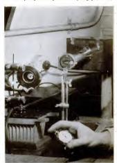
THE SPECTROGRAPH tests the absorbing power of a glass (center). Ultraviolet from spark (left) passes through test glass and registers on film (right).
