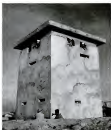
BLOCKHOUSES like this at Moncay, on Chinese border, stud countryside. Made of old brick and barely cemented over, they are highly vulnerable to shellfire.
